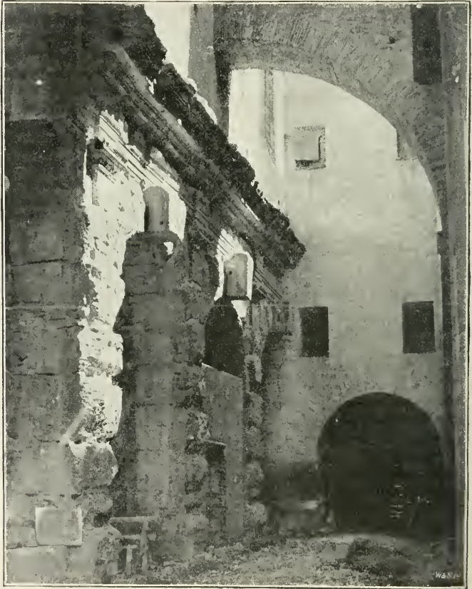
Fig. 133. — The Substructures of the Claudium, West Side.
