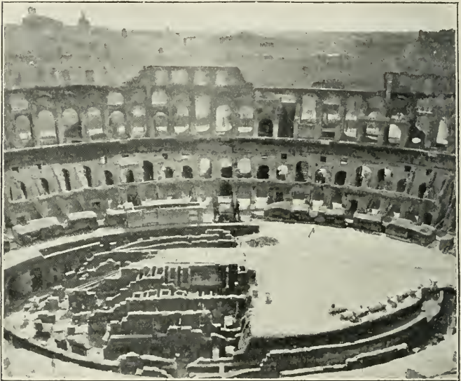
Fig. 141. — The Shell of the Coliseum after the Collapse of the Western Arcades.
