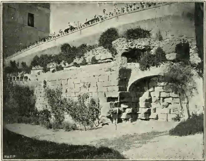
Fig. 114. — Remains of the Platform of the Capitoli-um in the Garden of the Caffarelli Palace.
