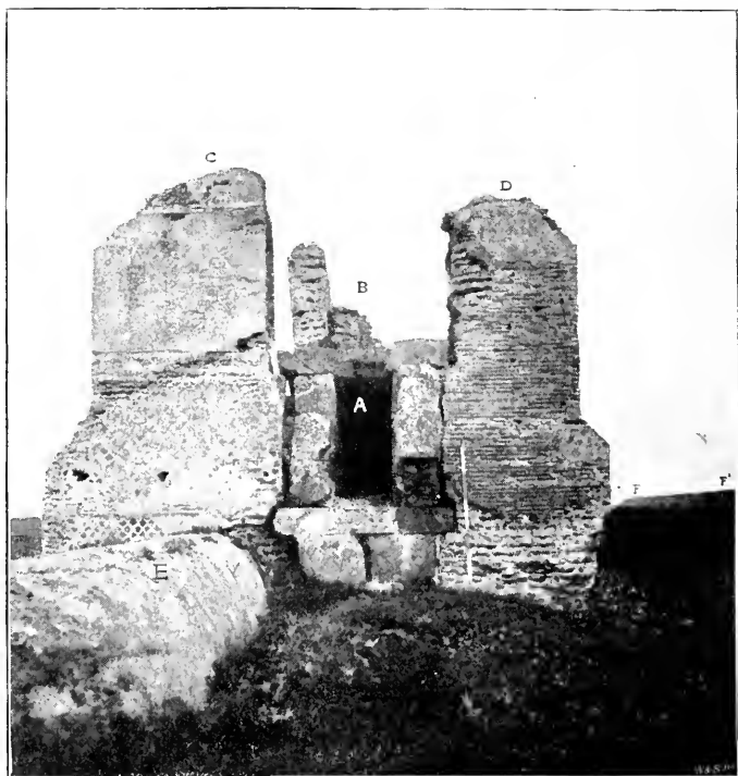
Fig. 22. — The Aqueducts at Roma Vecchia.
