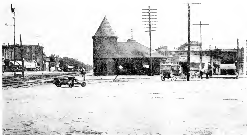
B. & O. STATION, NORTH VERNON, JENNINGS COUNTY
