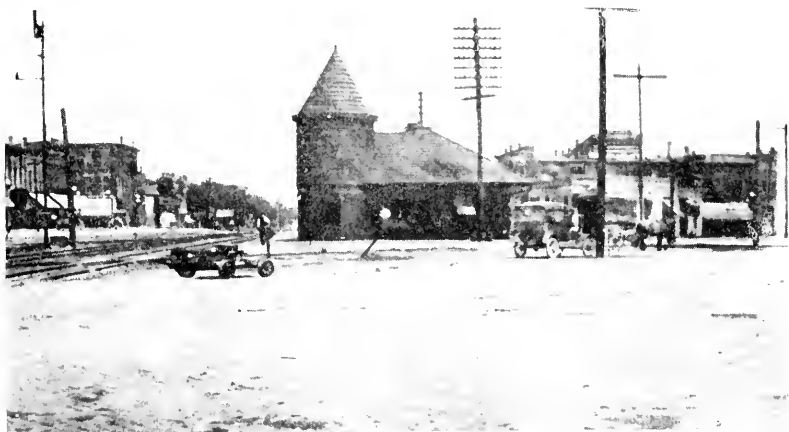
B. & O. STATION, NORTH VERNON, JENNINGS COUNTY
