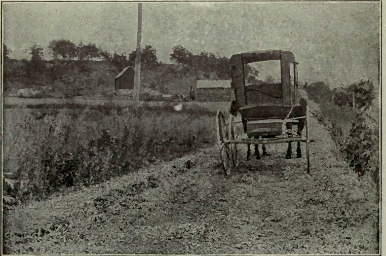
Fig. 2. Sand road freshly covered with straw
