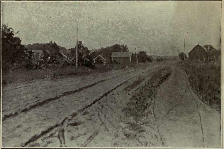
Fig. 1. Sand road showing effect of removal of trees and brush and consequent drying out of the road.
