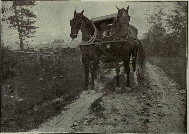
Fig. 2. Gravel road in Washington county with sod and coarse gravel heaped in the center with the road machine.
