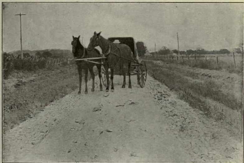
Fig. 2. Crushed stone road which has been compacted by the travel. Notice the loose character of the stones outside the beaten track.
