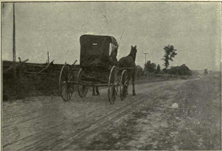
Fig. 1. A flat-topped clay road in Clark county. The ruts appearing in the picture are wheel tracks in a thick layer of dust.
