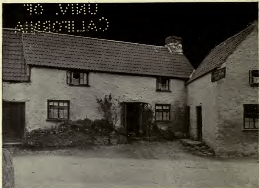
FIG. 11.—House with earth (forming flower-beds) banked against the front wall and contributing to its dampness.
