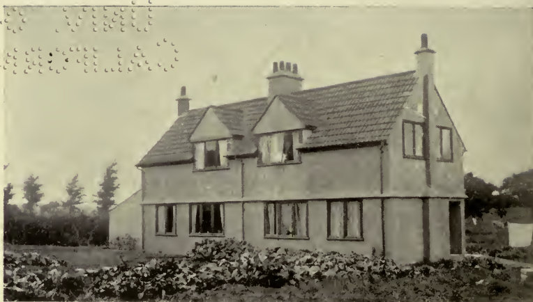
FIG. 27.—Pair of cottages at Winscombe constructed of concrete blocks. Built under the Co-operative Housing Scheme, described on page 241.
