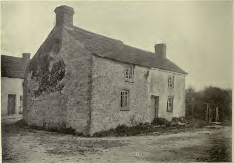
FIG. 7.—House built on odd piece of land with road front and back. There is a tiny piece of garden at one end, but insufficient for refuse and excreta disposal. This constitutes a great difficulty with houses built without land round. This particular house is very defective (there are no openings on the other side) and unfit, and was closed about a year before the photograph was taken.
