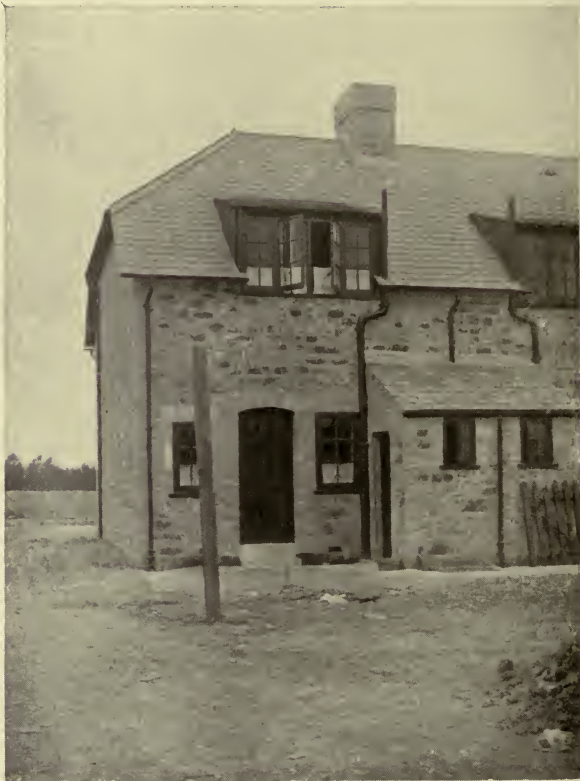
FIG. 32.—Martock houses. Back view of one of the end houses.
