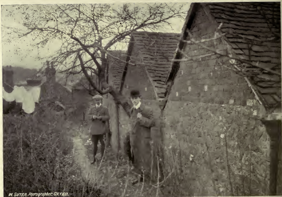
FIG. 20.—This illustration, and Figs. 21 and 22, illustrate the possibility of extensively improving existing cottages in suitable cases. This block of ten cottages in Oxted, Surrey, were originally without through ventilation, constantly damp, and insanitary.
