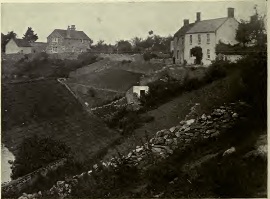
FIG. 10.—House built on sloping ground. The rain runs down the slopes and soaks up into the outside walls. To face page 63.
