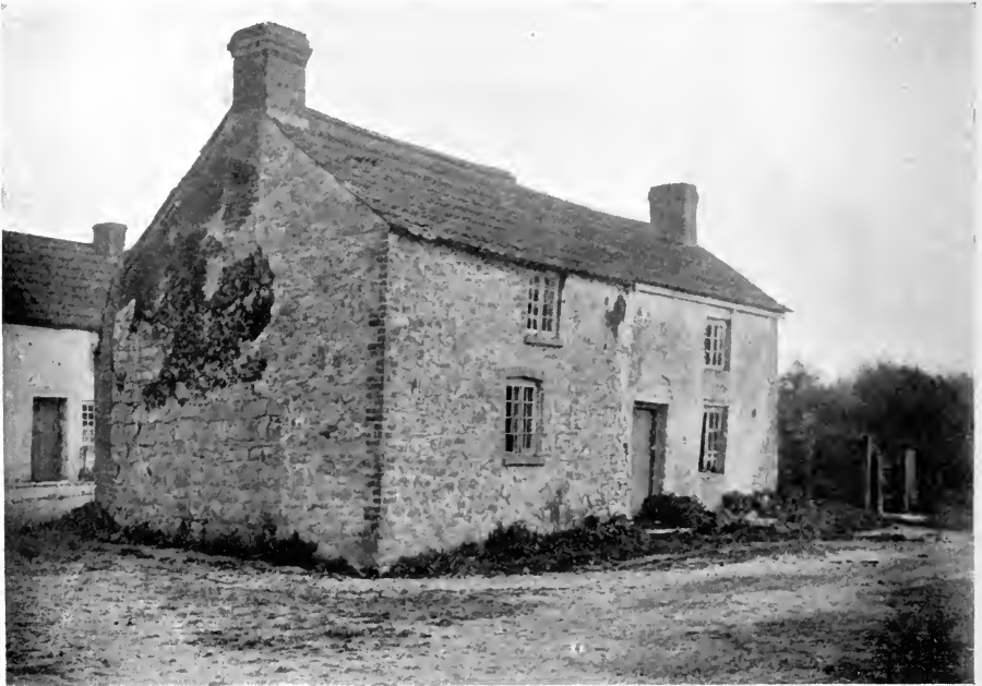
FIG. 7.—House built on odd piece of land with road front and back. There is a tiny piece of garden at one end, but insufficient for refuse and excreta disposal. This constitutes a great difficulty with houses built without land round. This particular house is very defective (there are no openings on the other side) and unfit, and was closed about a year before the photograph was taken. To face page 59.
