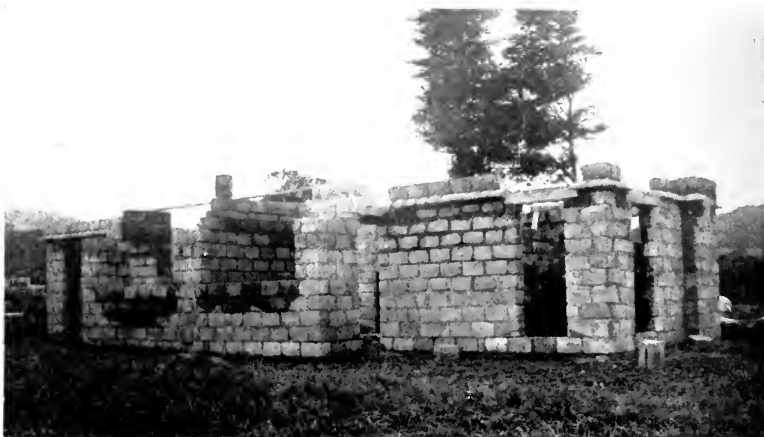
FIG. 28.—Pair of cottages similar to those in Fig. 27, in course of erection.
