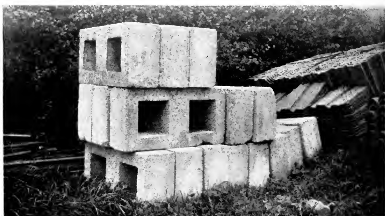
FIG. 29.—Concrete blocks used in construction of the houses shown in Fig. 27 and Fig. 28.
