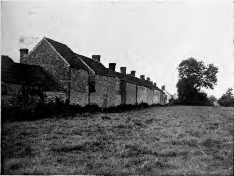
FIG. 4.—Back view of same row of cottages as Fig. 3. Note the absence of through ventilation and of shutting.
