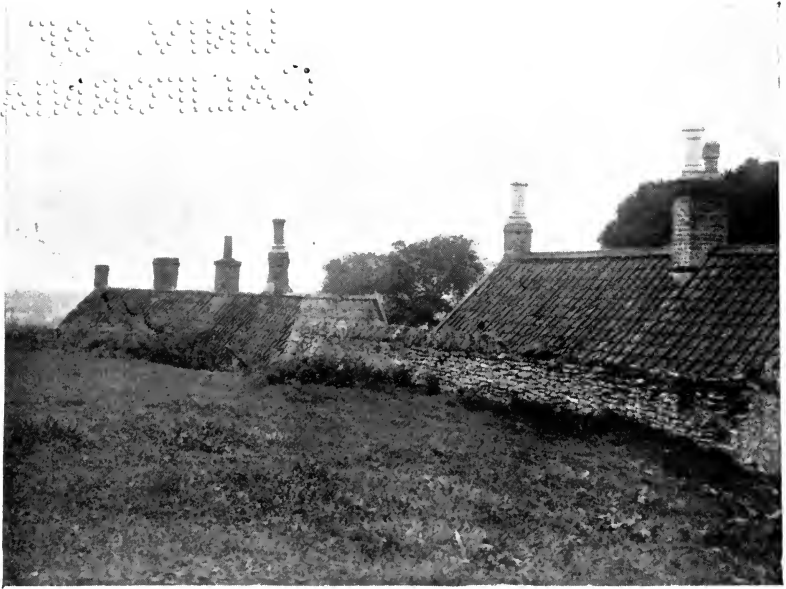
FIG. 8.—To illustrate houses built on lower ground and without air space at the rear.
