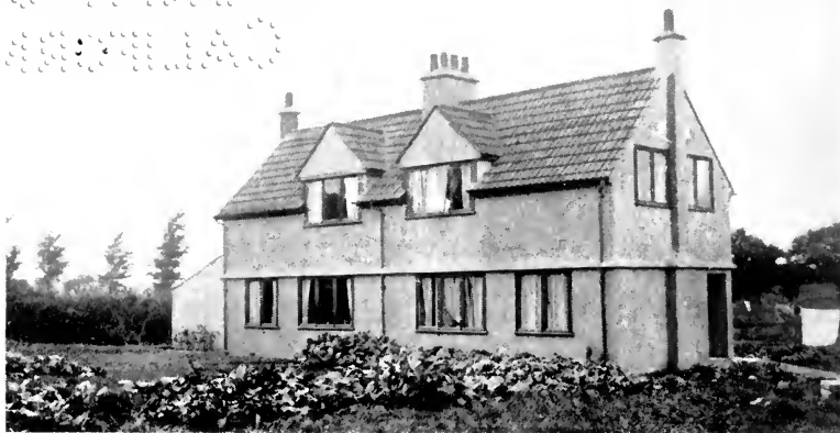
FIG. 27.—Pair of cottages at Winscombe constructed of concrete blocks. Built under the Co-operative Housing Scheme, described on page 241.
