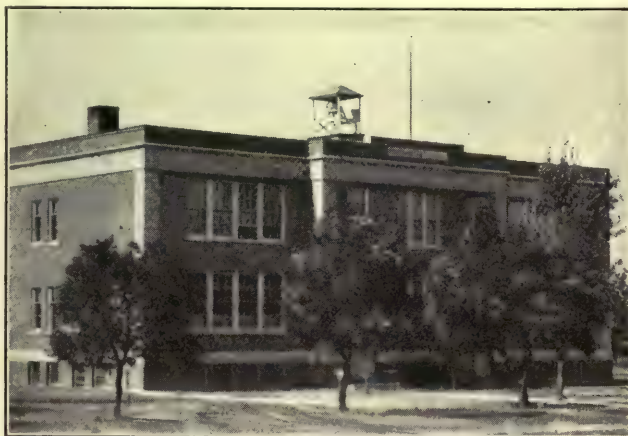
A substantial and well-planned building
