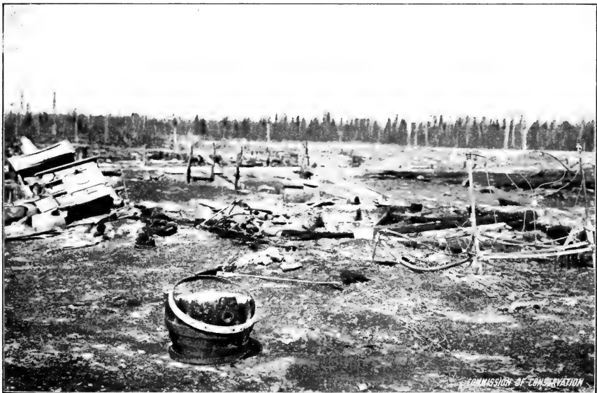
REMAINS OF SETTLER'S HOME After forest fire in the "Clay Belt" of Northern Ontario, 1916
