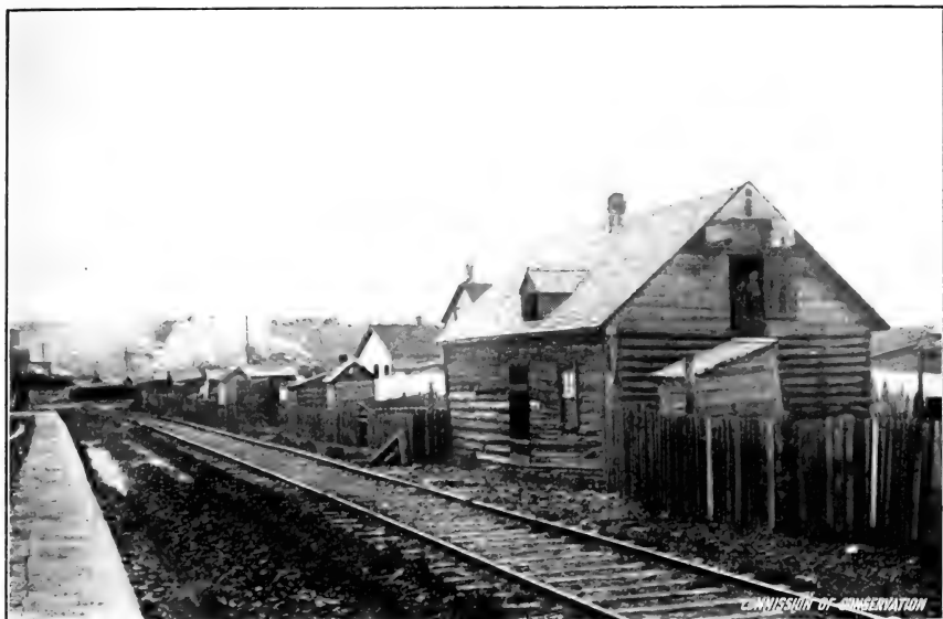
UGLY AND DANGEROUS SLUM CONDITIONS ADJOINING A RAILWAY
