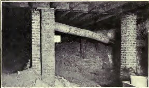
What a visit to the basement revealed
