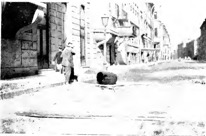
MR. WELLS DISCOVERS A STREET UNDER REPAIR.
