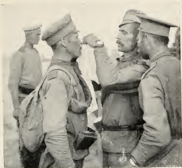
Respirator drill in the trenches.
