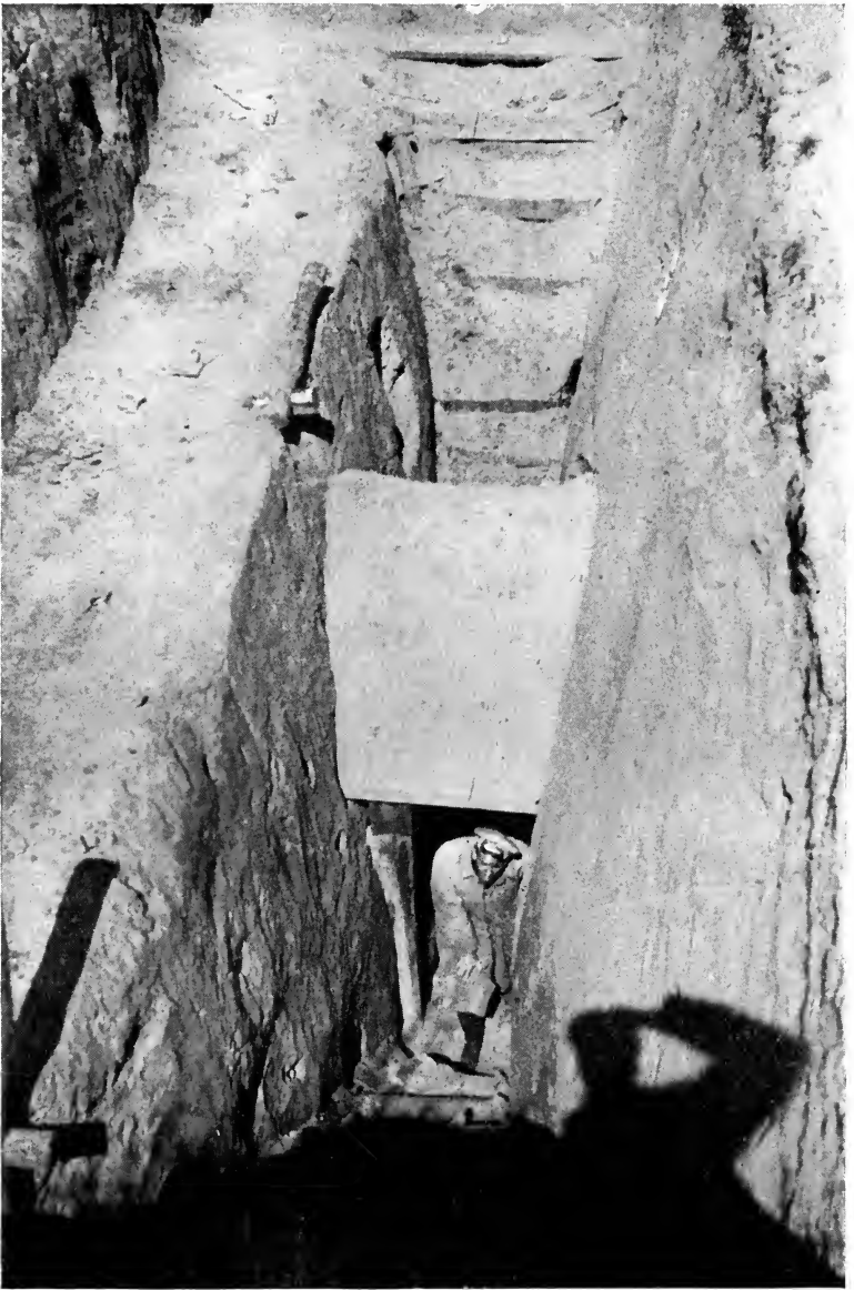
AN AUSTRIAN SHELTER NEARLY THIRTY FEET BELOW GROUND SHOWING ENTRANCE TO AN UNDERGROUND CAVERN PROVIDED FOR OFFICERS.
