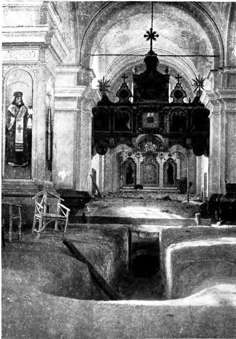
AUSTRIAN TRENCH DUG IN DUBNO CHURCH.
