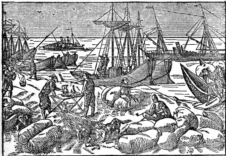
PREPARING TO BRIDGE THE DANUBE FROM WIDDIN TO KALAFAT.
