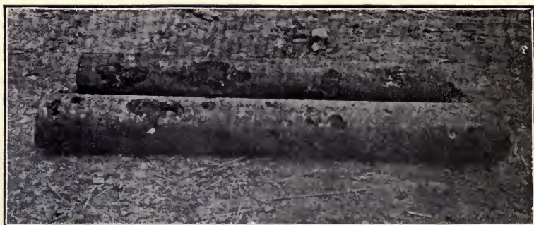
FIG. 84.—Effect of electrolysis on 6-inch cast-iron pipes, Kansas City, Mo.
