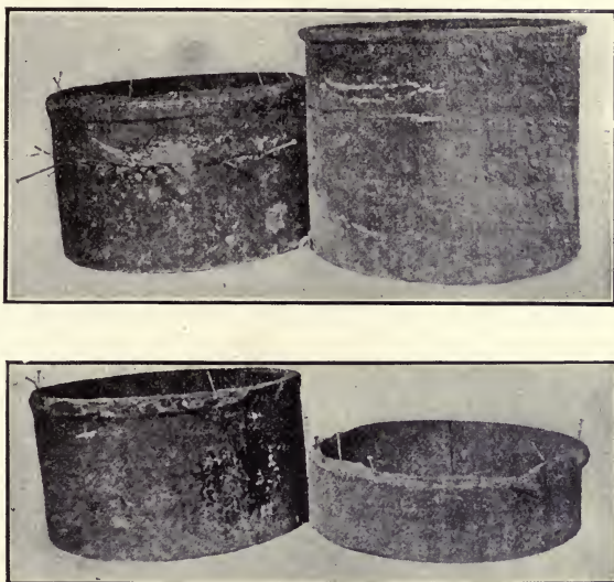
FIG. 79.—16-inch cast-iron suction pipes (page 380).
