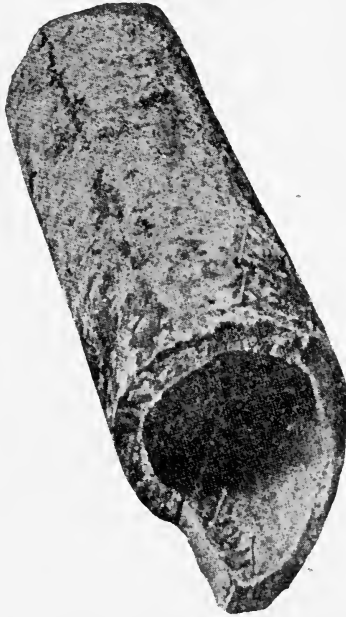
FIG. 77.—Electrolytical pittings no inside and outside of 4-inch cast-iron water-pipe.
