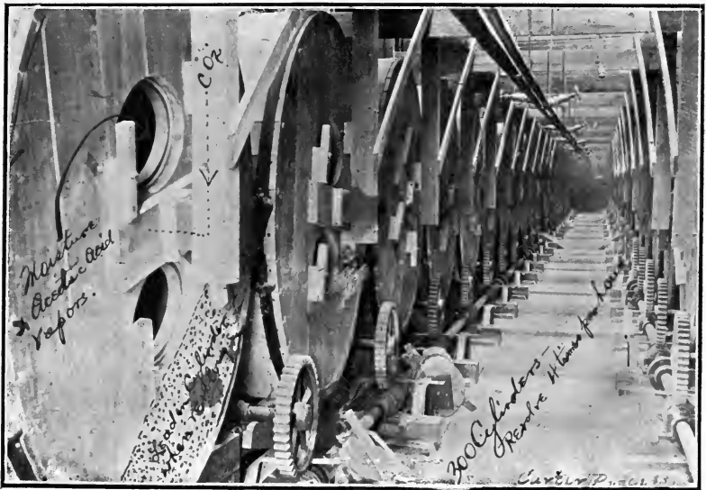
FIG. 13.—The Carter process for manufacturing white lead.
