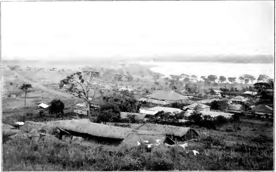
GENERAL VIEW OF ENTEBBE.
