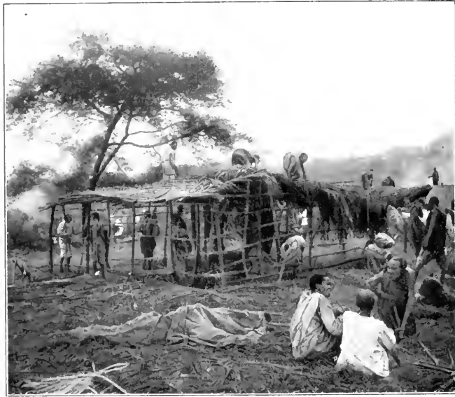
BUILDING SHEDS, UGANDA.
