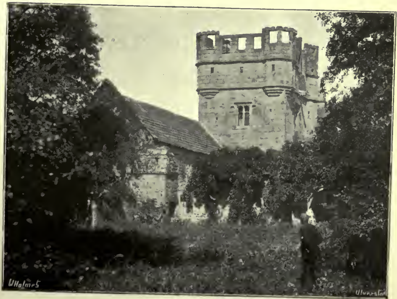
MORTHAM TOWER FROM THE NORTH.
