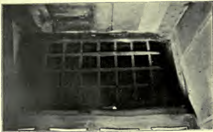
IRON BARRED GATE.
