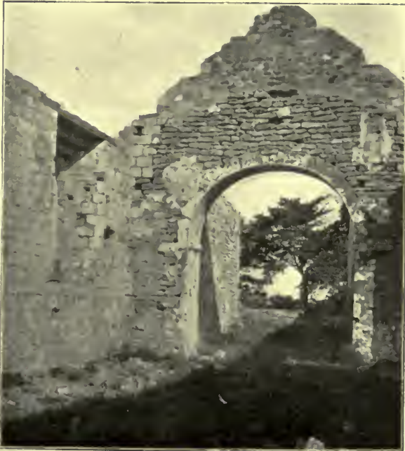
CHANCEL ARCH, GRINDON CHURCH, FROM THE WEST.
