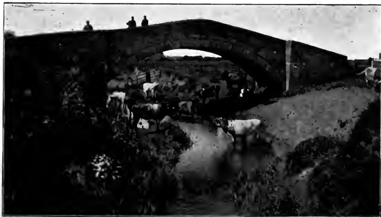
BELLASIS BRIDGE. (From a photograph by Mr. P. Brewis.)
