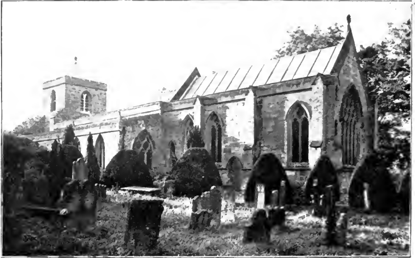
ST. MARY'S CHURCH, MORPETH. From the South East.
