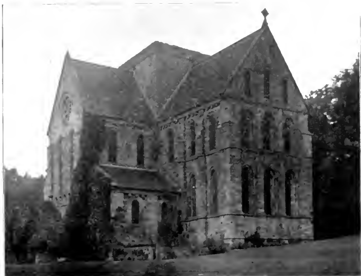
BRINKBURN PRIORY FROM S.E. (From a photograph by Mr. Joseph Oswald.)
