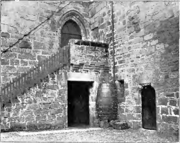
DOORWAY TO HALL.
