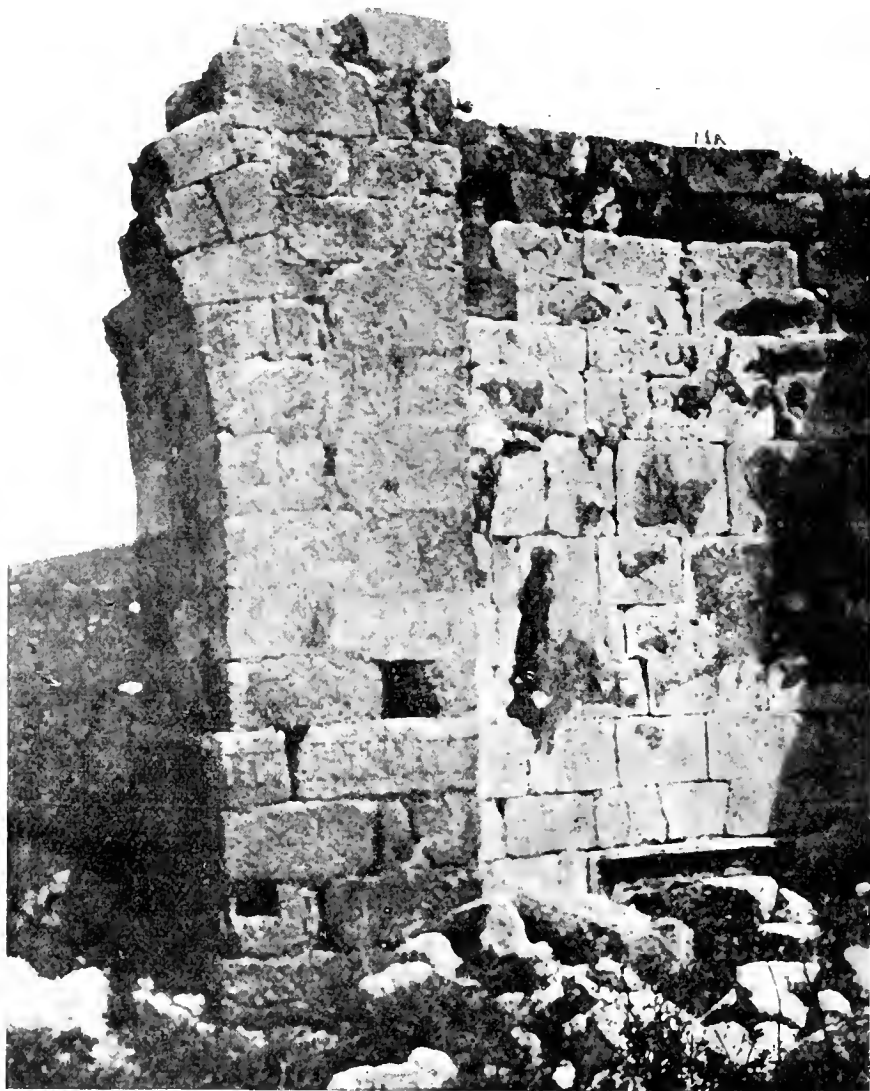
Fig. 5. — Spring of north western arch of nave northern basilica. Budrum.
