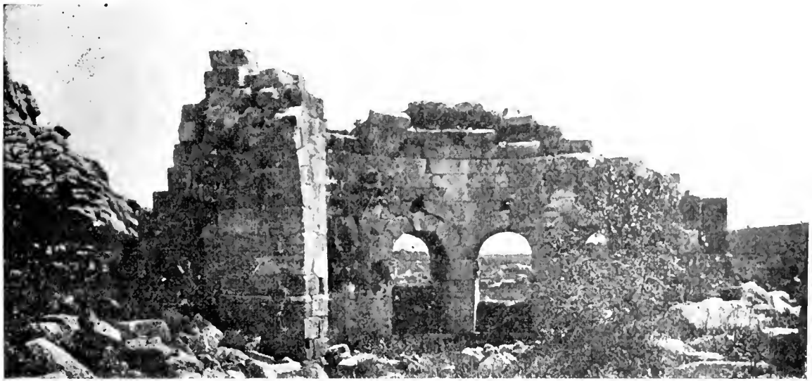
Fig. 6. — Interior of apse, northern basilica. Budrum.
