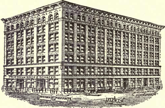
The Mallinckrodt Building, St. Louis, Mo., Contains 300 H. P. Heine Boilers.
