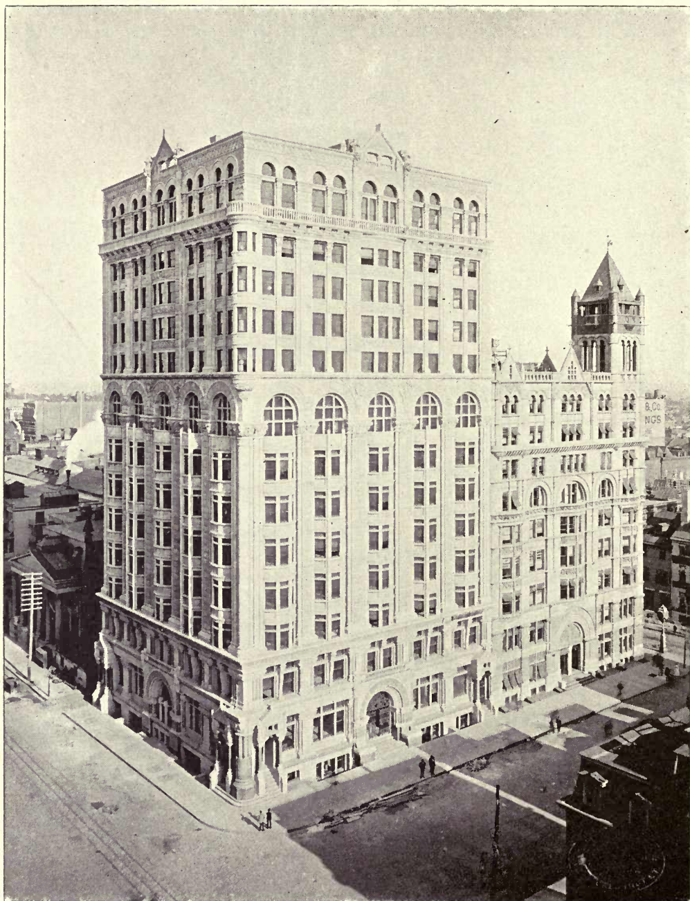
The Betz Building, PHILADELPHIA, PA. Contains 500 H. P. Heine Boilers.
