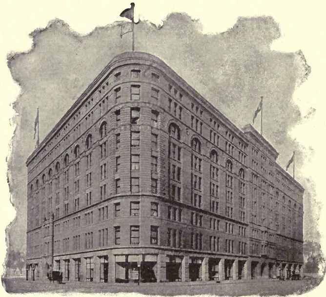
Brown Palace Hotel, Denver, Col. Heat and Power from 520 H. P. of Heine Boilers.
