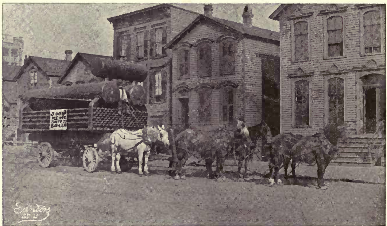
300 H. P. Heine Boiler being moved.
