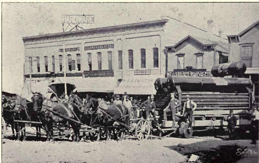
250 H. P. Heine Boiler "en route."
