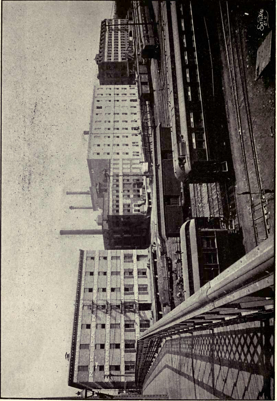
N. K. Fairbank & Co.'s Factories, CHICAGO, ILL., Contain 1500 H. P. of Heine Boilers.
