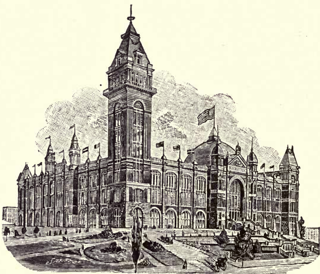
Minneapolis Industrial Exposition Building, Minneapolis, Minn., With Heine Boiler Plant of 1000 H. P.
