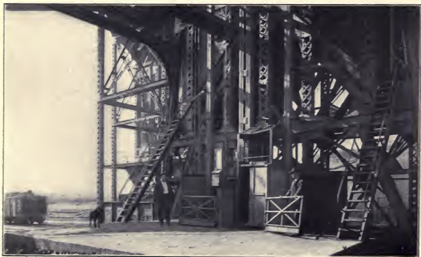
LEVEL CONCRETE PLATFORM AND SAFETY GATES AT THE OLIVER MINING COMPANY'S SHAFT
