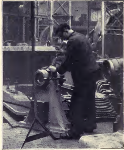
MOVABLE SCREEN TO PROTECT OTHER WORKMEN AND PASSERS-BY FROM FLYING CHIPS OF METAL. ALLGEMEINE ELEKTRICITAETS GESELLSCHAFT
