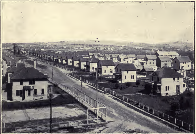
WORKMEN'S DWELLINGS IN ONE OF THE TOWNS OF THE OLIVER MINING COMPANY
