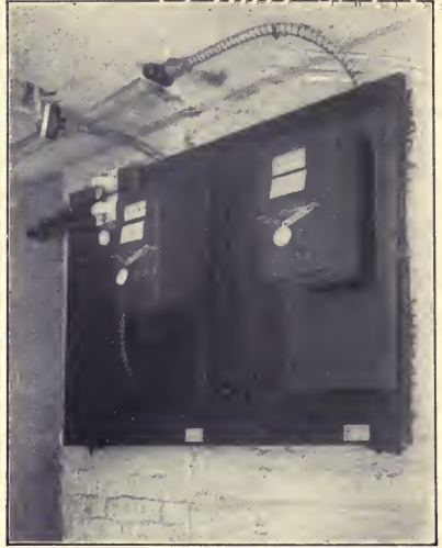
SEALED CUT-OUT; FUSES AND WIRES INCASED IN PORCELAIN OR METAL
