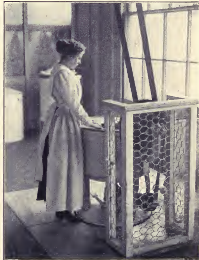
GUARDS OVER BELTS IN LAUNDRY. NATIONAL CASH REGISTER COMPANY
