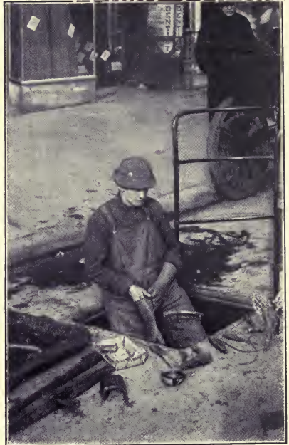
THE NEW YORK EDISON COMPANY'S GUARDS FOR MANHOLE IN A CITY STREET
