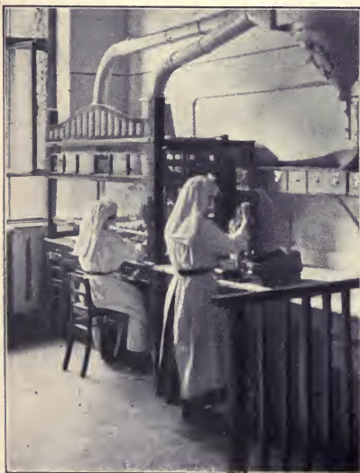
HOODED CAPS AND EXHAUSTS FOR PREVENTING WORKERS FROM INHALING DUST. FRIED. BEYER, LEVERKÜSEN
