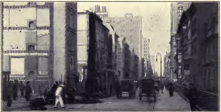
UNSIGHTLY AND DANGEROUS STREET OBSTRUCTIONS
