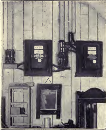
OLD-STYLE INSTALLATION—WIRING AND CUT-OUTS EXPOSED AND MOUNTED ON A WOODEN PARTITION
