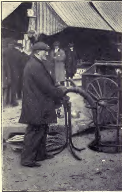
THE NEW YORK EDISON COMPANY'S GUARDS FOR MANHOLE IN A CITY STREET
