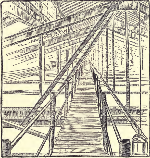
RAILED WALK FOR ARC LAMP TRIMMERS
