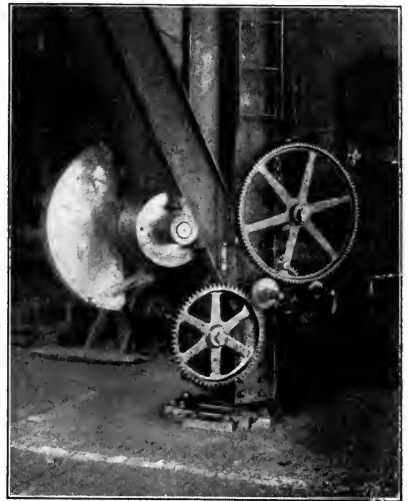
GEAR COVERS ON JIB CRANE REMOVED
