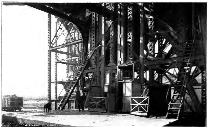
LEVEL CONCRETE PLATFORM AND SAFETY GATES AT THE OLIVER MINING COMPANY'S SHAFT
