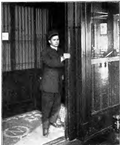
DEVICE FOR ILLUMINATING THRESHOLDS AS ELEVATOR APPROACHES EACH FLOOR AT THE NATIONAL CASH REGISTER COMPANY
