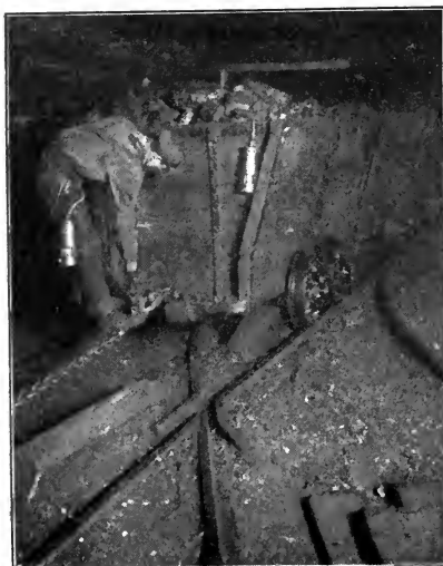
OLD METHOD OF UNCOUPLING LOADED CARS AT SHAFT BOTTOM
