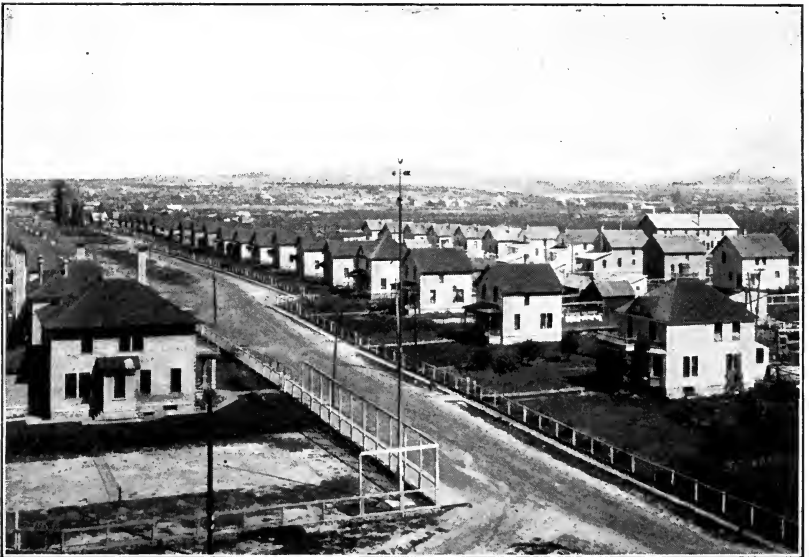
WORKMEN'S DWELLINGS IN ONE OF THE TOWNS OF THE OLIVER MINING COMPANY
