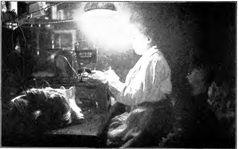
MORE LIGHT IN EYES THAN ON WORK. POOR DIFFUSION. WRONG LOCATION OF LAMP
