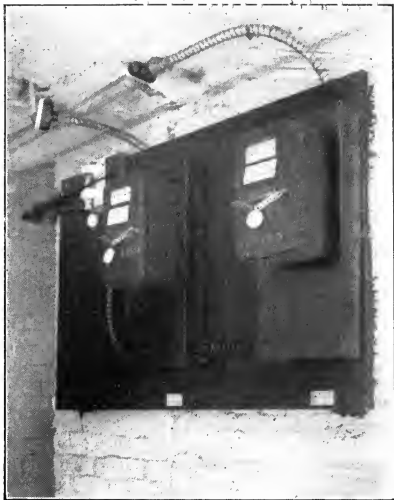
SEALED CUT-OUT; FUSES AND WIRES INCASED IN PORCELAIN OR METAL
