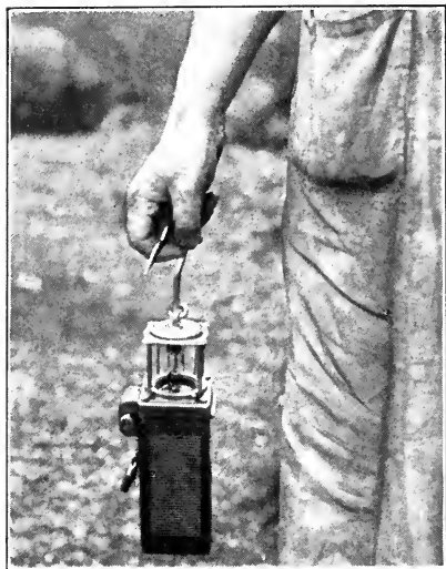
THE EDISON PORTABLE SAFETY LAMP FOR MINERS
