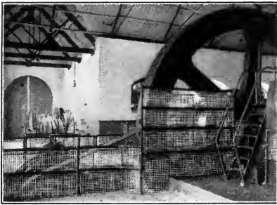
GUARDS AROUND FLY-WHEEL AND CONDENSER PUMP
