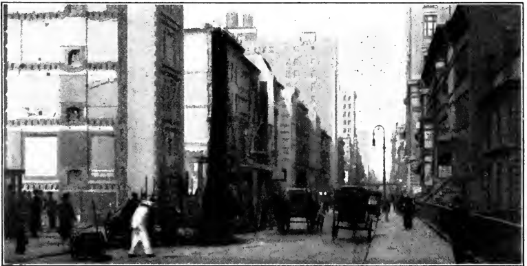
UNSIGHTLY AND DANGEROUS STREET OBSTRUCTIONS
