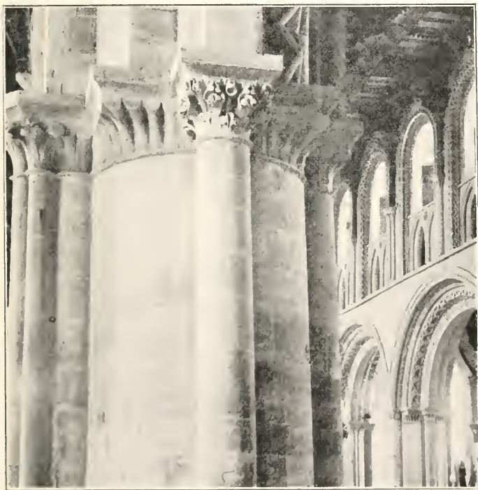
NORMAN SHAFT WITH RE-CARVED CAPITAL, EASTERN PIER IN S. NAVE ARCADE. (See p. 27.)
