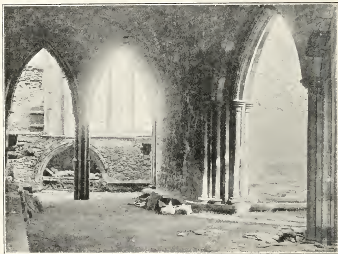
VIEW LOOKING W. IN ANTE-CHAPEL TO LADY CHAPEL.
