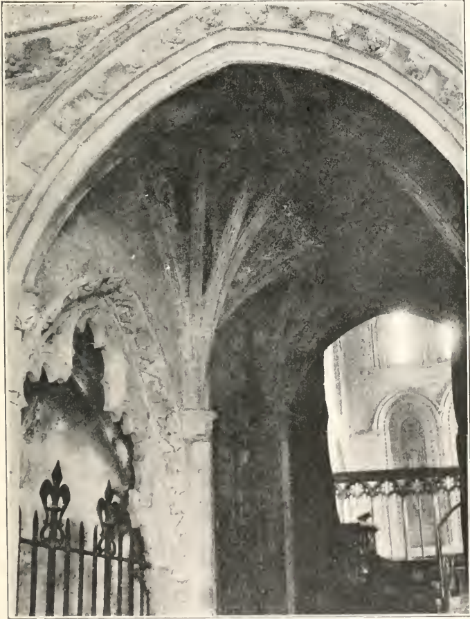
GROINING OF ROOD SCREEN, SHOWING THE FLYING RIBS.
