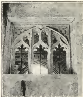
RECENTLY DISCOVERED WINDOW IN BISHOP VAUGHAN'S CHAPEL.
