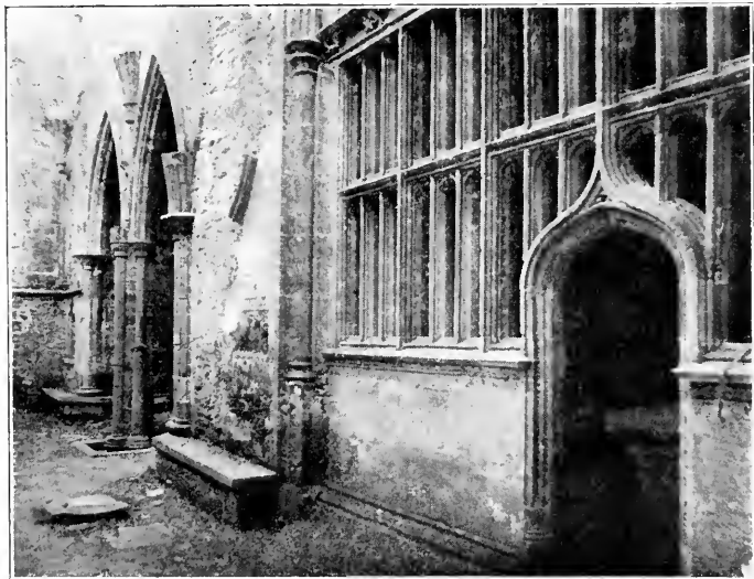
THE NORTH CHAPEL AISLE.
