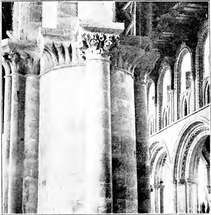
NORMAN CHURCH WITH RE-CARVED CAPITAL, EASTERN PIER IN S. NAVE, AR. ADL. (See p. 27.)
