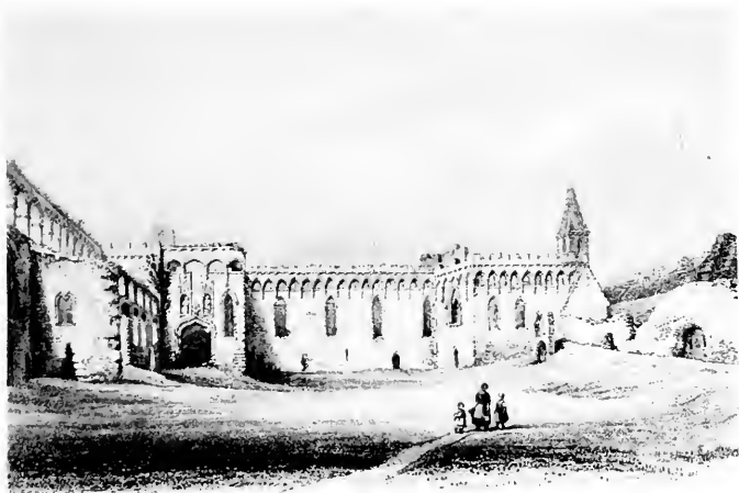
BISHOP'S PALACE: GENERAL VIEW OF COURTYARD LOOKING TOWARDS ENTRANCE TO GREAT HALL.
