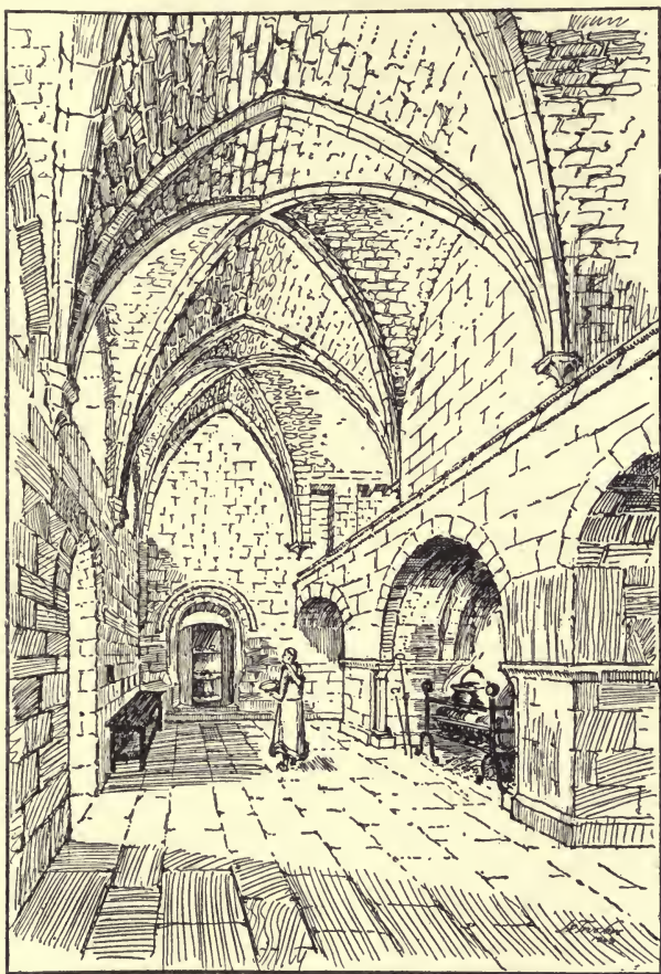
FOUNTAINS ABBEY. Restoration of the Kitchen
