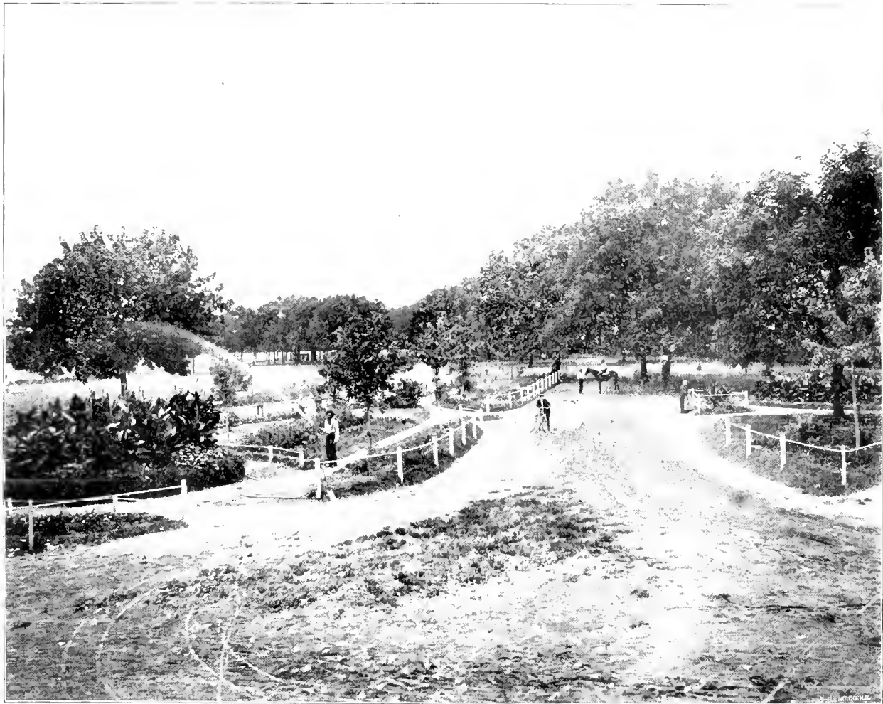
OAKDALE PARK AS VIEWED FROM MAIN ENTRANCE
