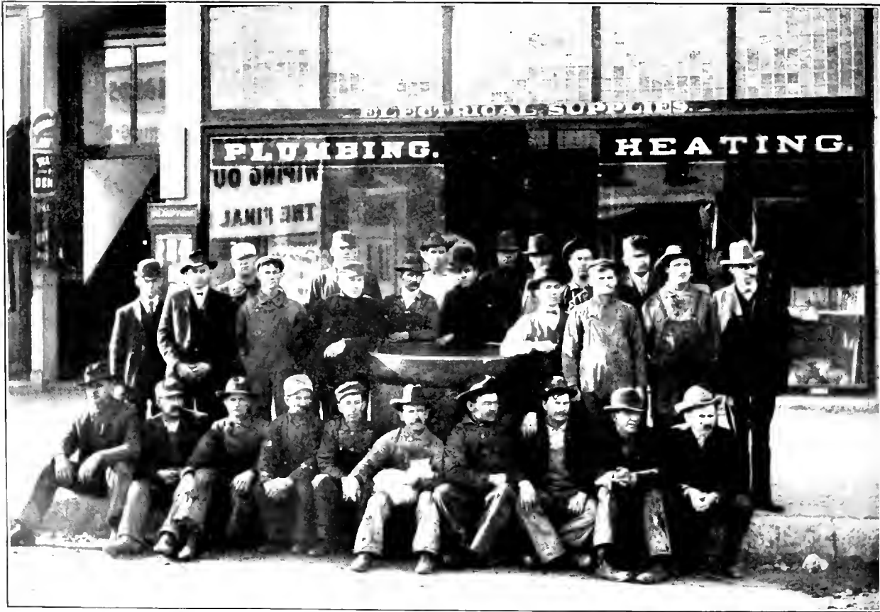
THE SALINA PLUMBING COMPANY Sanitary Plumbers Heating Engineers, Electricians, Tin and Sheet Metal Workers
