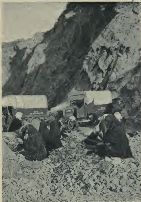
Macedonian "Ladies" breaking stones for road-making.
