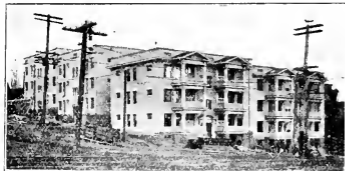
Brick Work on this Building Done by Us
