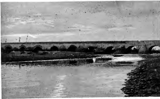
A BRIDGE OVER THE TENSIFT, MOROCCO CITY
