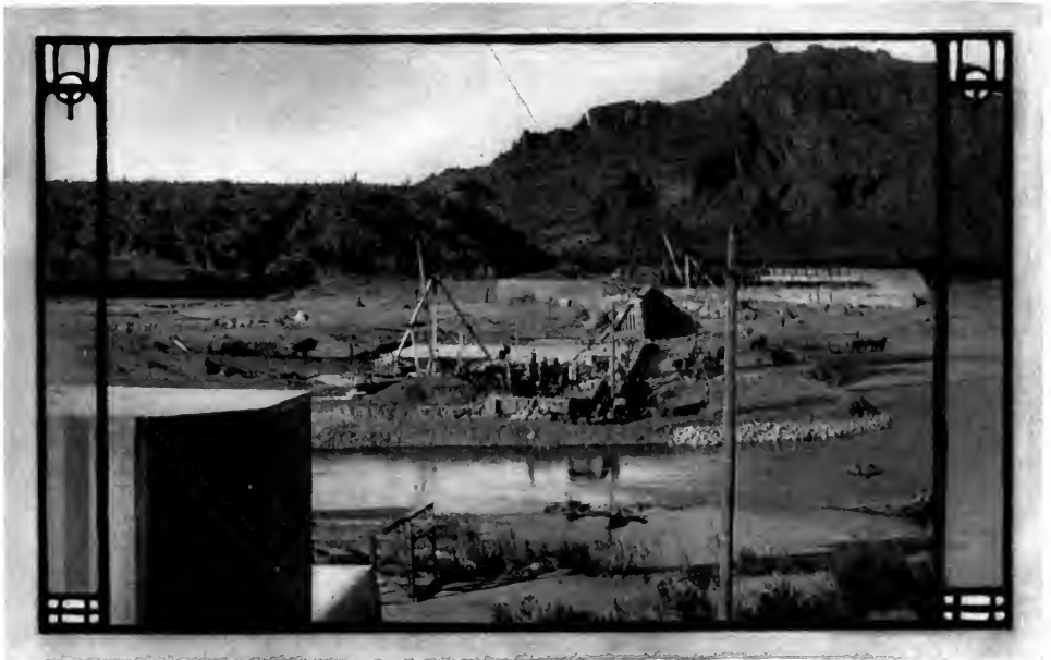
Constructing Granite Reef Division Dam
