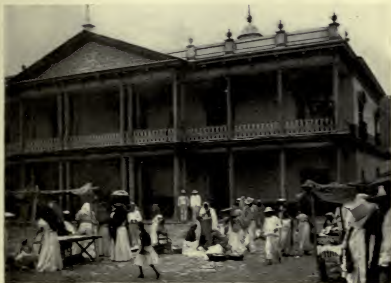
BARRACKS AT COJUTEPEQUE, DEPARTMENT OF CUSCATLÁN.
