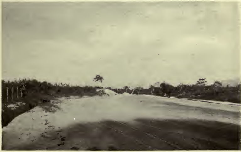
THE FAMOUS AVENIDA UNDER CONSTRUCTION.
