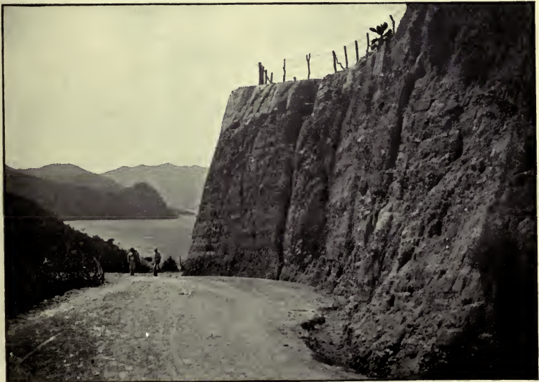
VIEWS ON NEW NATIONAL ROAD, BETWEEN SAN VICENTE AND ILOPANGO.
