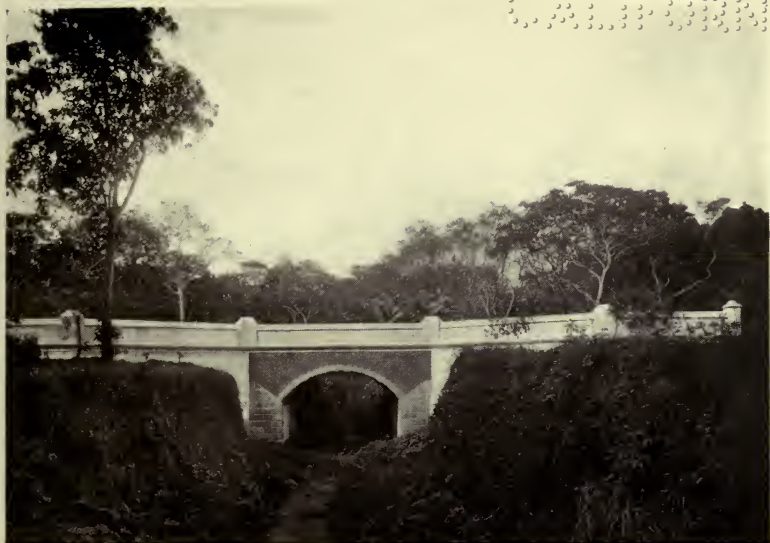
SIDE VIEW OF "EL ROTULO" BRIDGE
