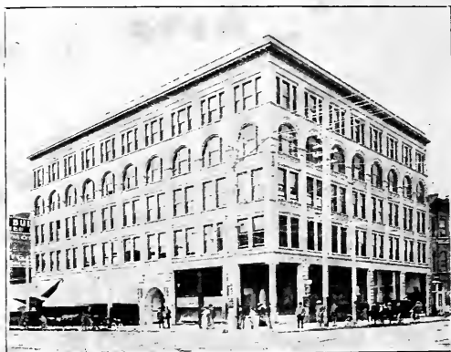
GRANGER BLOCK, FIFTH STREET, S. W. CORNER D STREET.
