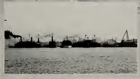
A busy day on the waterfront, The Bethlehem plant, San Francisco.
