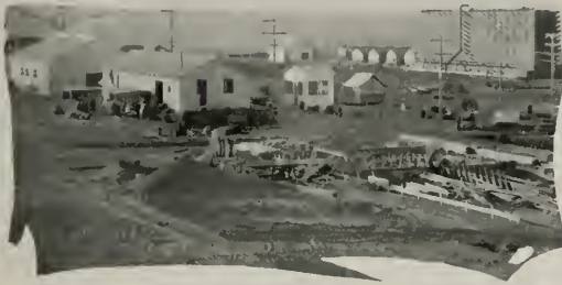
Beginning of Million-Dollar Compressor Plant, Kettleman Hills
