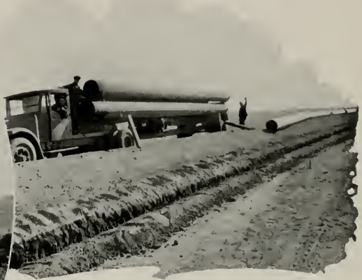
Laying out pipe along right of way, valley line
