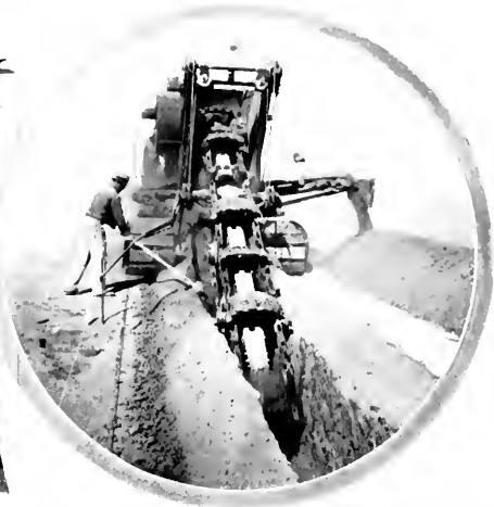
Excavating for pipe line
