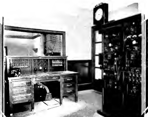
Control Booth of KPO showing Control Desk and section of Speech Input Panel.
