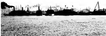
A busy day on the waterfront. The Bethlehem plant, San Francisco.
