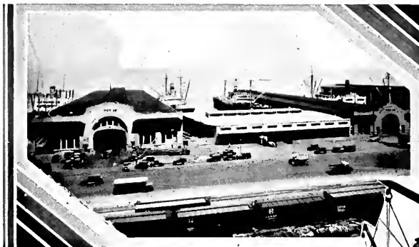
Above, "Less than carload lots" sheds constructed at American-Hawaiian Steamship Company pier to avoid congestion of freight and to speed up loading.
