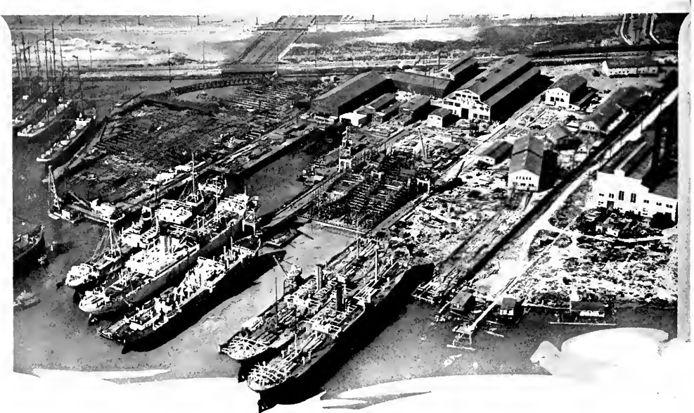
Four large ships under construction in a San Francisco Bay plant. In the foreground, two nearing completion. The two in the center are in the early stages of construction.
