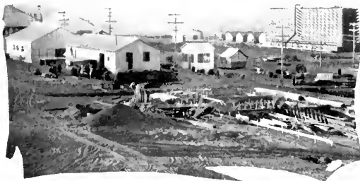
Beginning of Million-Dollar Compressor Plant, Kettleman Hills
