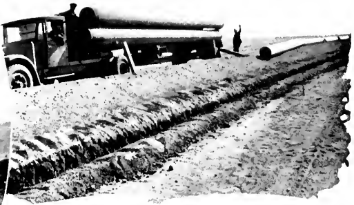
Laying out pipe along right of way, valley line
