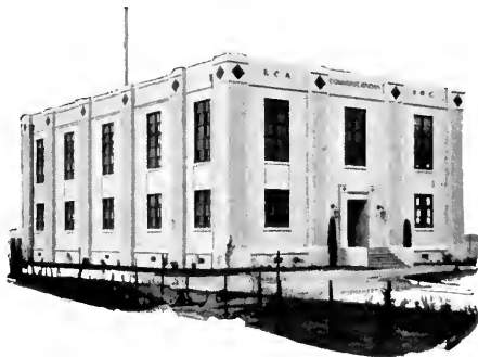
RCA Communications, Inc., new power house at Bolinas, Calif., which houses many short wave transmitters for direct communication with Hawaii, Japan, China, The Philippines, Dutch East Indies, French Indo-China and other countries.
