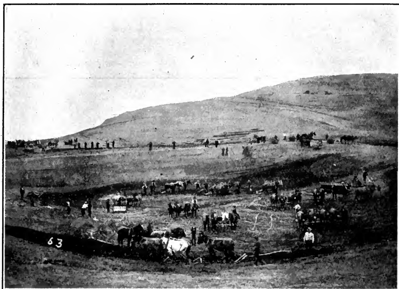
Excavating the Site for the Twin Peaks Reservoir.
