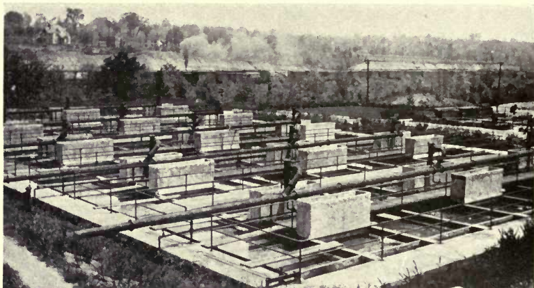
FITCHBURG, MASSACHUSETTS A large Imhoff tank sewage treatment plant
