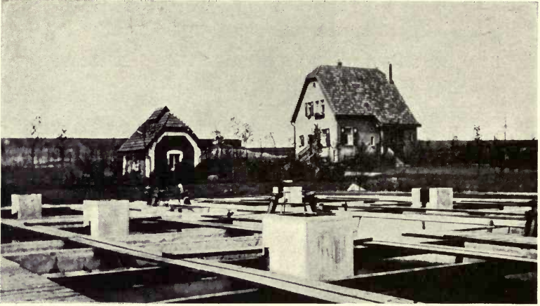
ESSEN, GERMANY Imhoff tank sewage treatment plant
