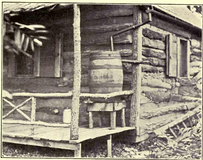
FIG. 14.—AN INEXPENSIVE AND SANITARY METHOD FOR COLLECTING RAIN-WATER.
