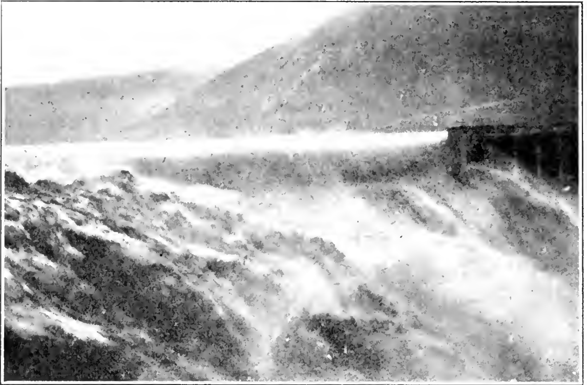
FIG. 2.—San Dieguito River near San Diego. Spillway of Lake Hodges, flood of 10,000 second-feet.
