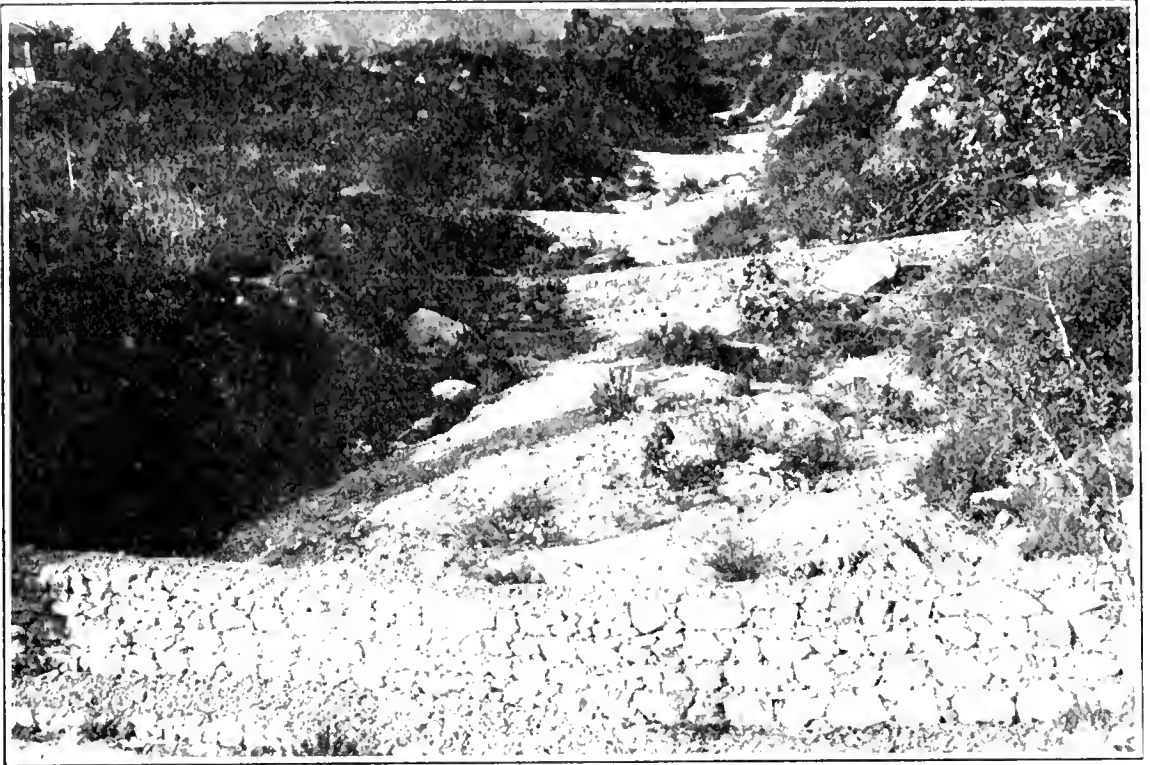
FIG. 27—Typical check dam construction.
