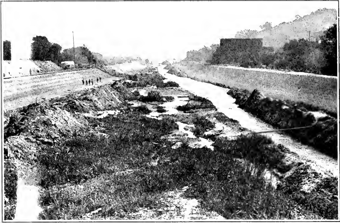
FIG. 23—Los Angeles River near Universal City. Four-inch rock and wire mattress.
