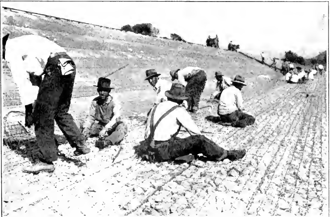
FIG. 22—Rock and wire mattress. Sewing mat with tie wires.
