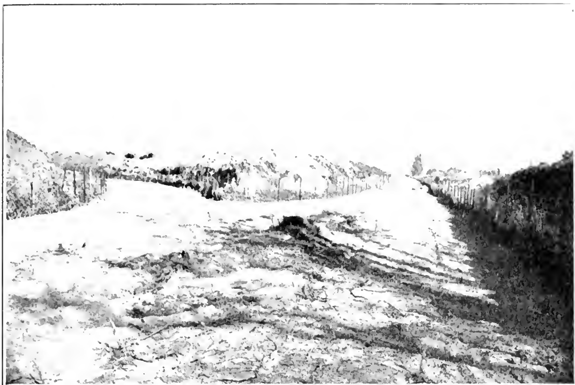
FIG. 9—Channel Control. Single pipe and wire mesh, Junction San Dimas and Big Dalton Wash.
