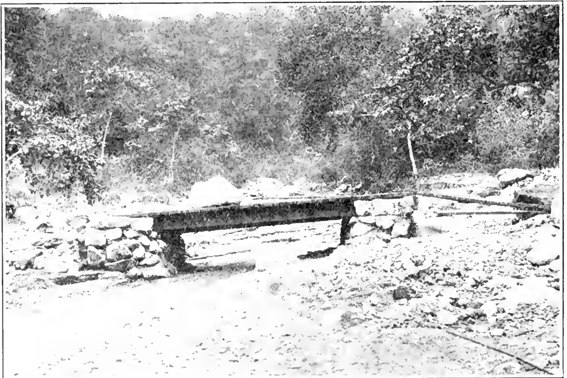
FIG. 4—Sawpit Canyon near Monrovia. Rock transported onto bridge by flood of April 7, 1925.
