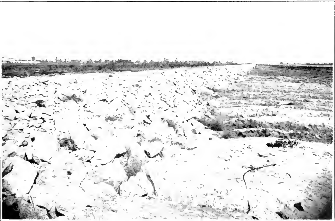
FIG. 18—Channel Control. Long Beach Channel north of Anaheim Bridge, showing riprap.
