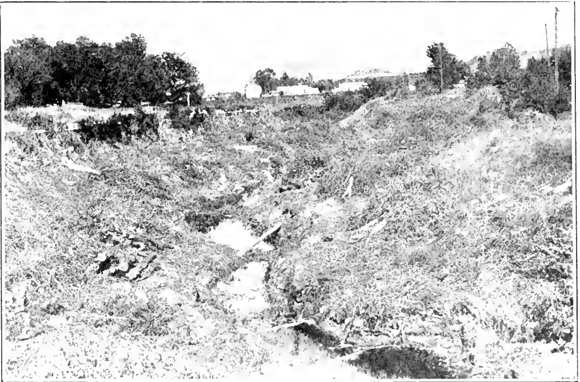
FIG. 36.—Los Angeles River. Channel clearing.
