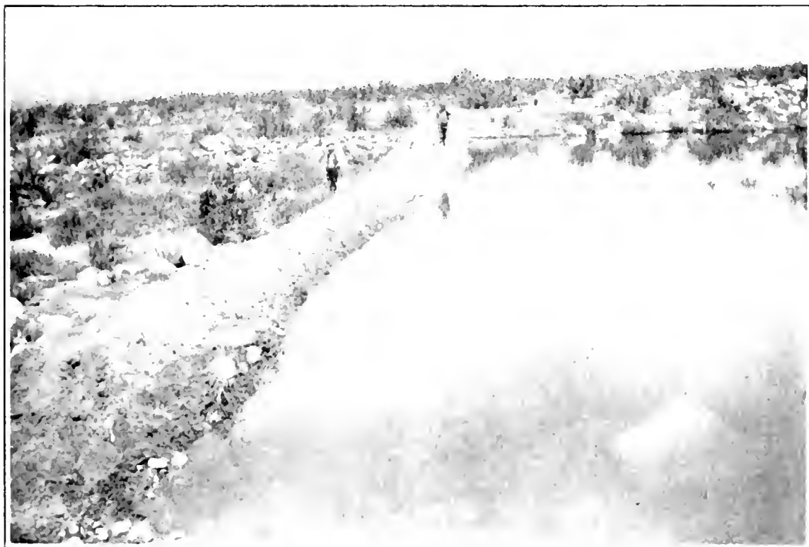
FIG. 42—Tri-Counties Works on Santa Ana River. A settling basin.
