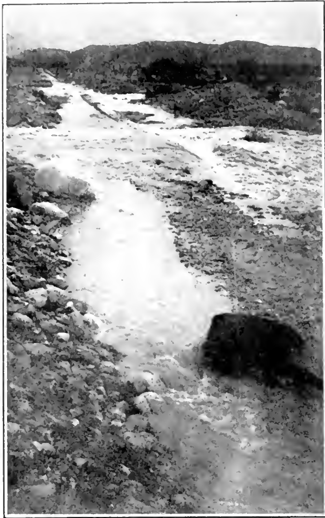
FIG. 40—Lytle Creek spreading and diversion dam. Flood on April 6, 1926.
