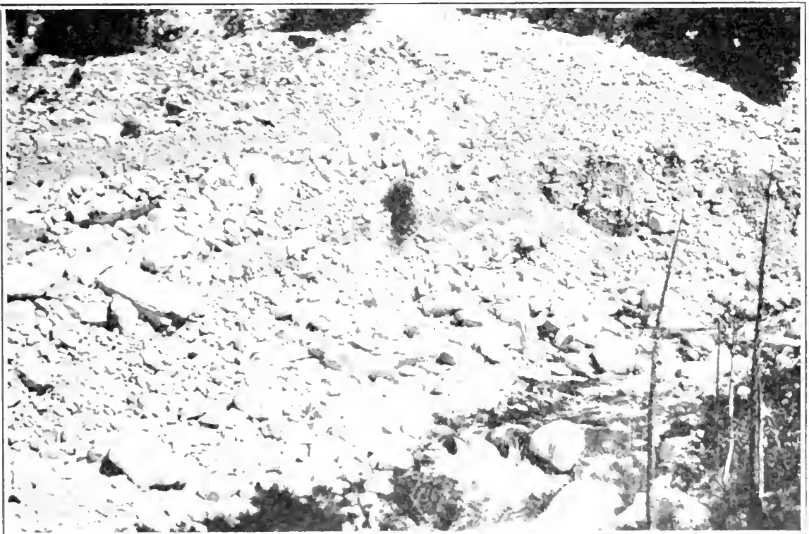
FIG. 6. Remnant of natural dam on Bear Creek at former Slide Lake, caused by debris carried by Slide Creek, a side canyon. The dam was washed out by flood of February, 1927.
