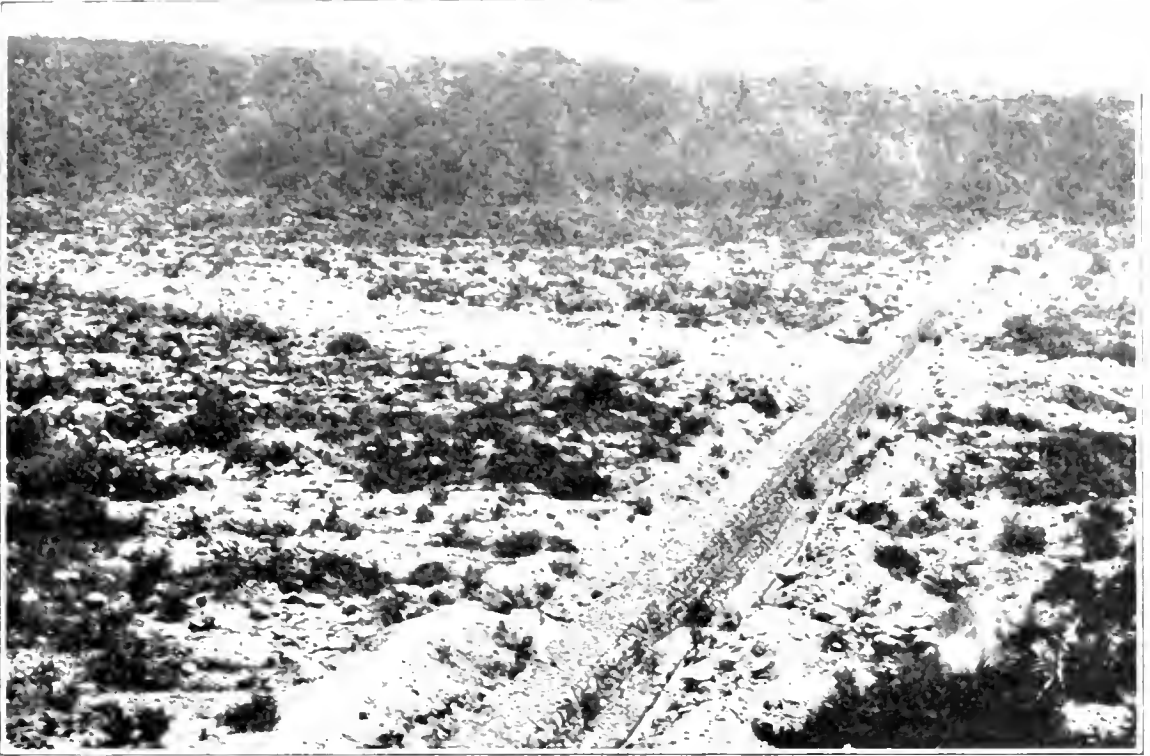
FIG. 37.—Cucamonga Water Company. Spreading dam on Cucamonga Creek. This dam is at right angles to the stream, and is the middle cross wall of the system.
