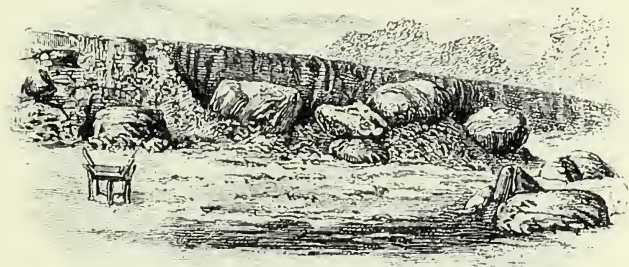
FIG. 83.—Section of Boulder-Clay, Craiglockhart Hill, Edinburgh. Exposed when the foundations of the Hydropathic Establishment were being dug out.
