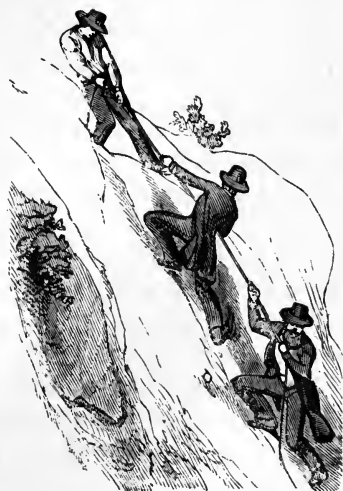
ASCENDING THE LOWER DOME.
