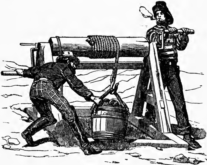
SINKING A SHAFT.
