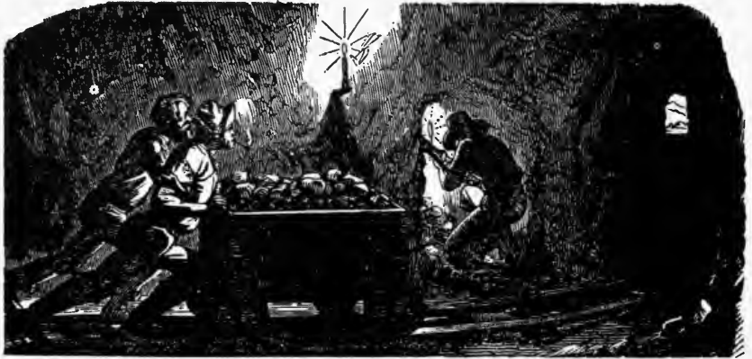
RUNNING A TUNNEL.
