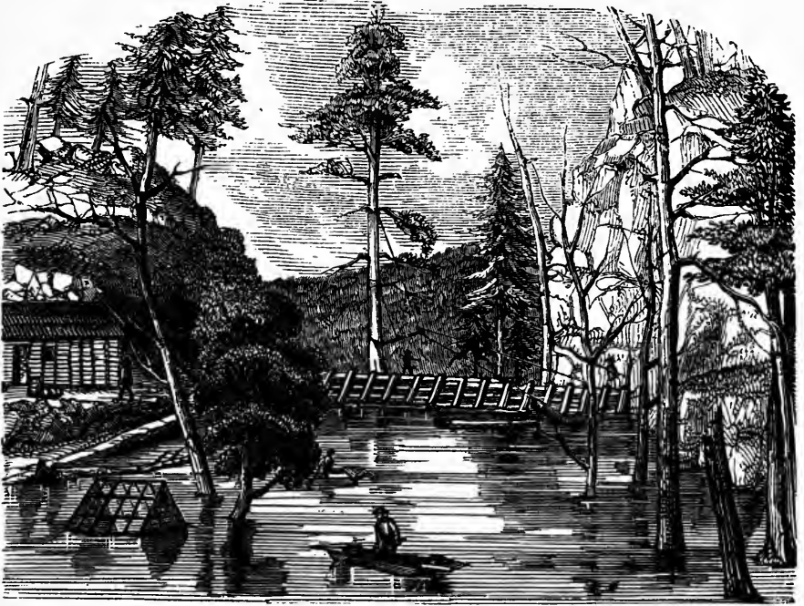
RESERVOIR OF THE TUOLUMNE COUNTY WATER COMPANY, AT STRAWBERRY FLAT.
