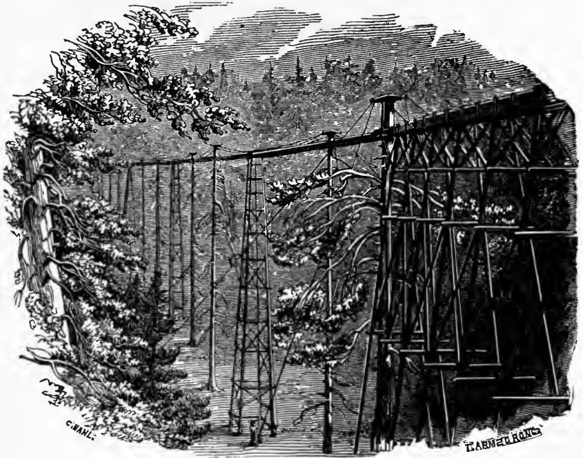
SUSPENSION FLUME ACROSS BRANDY GULCH.
