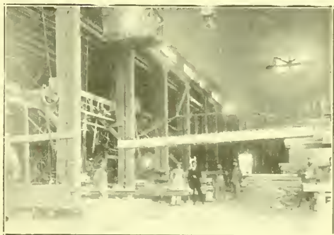
Interior of Stone Mill
