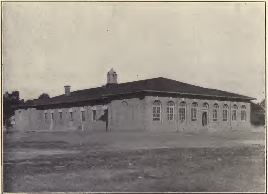
Rear view of eight-room Grammar School at Artesia.
