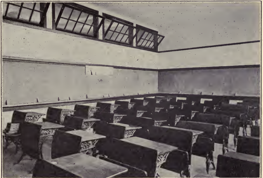
Interior of typical classroom, looking toward the ventilating transoms that open into the corridor.
