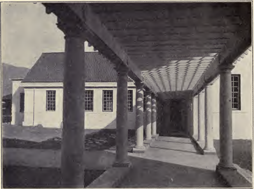
Monrovia Polytechnic High School, showing beautiful cloister between the main building and the Manual Arts Building.
