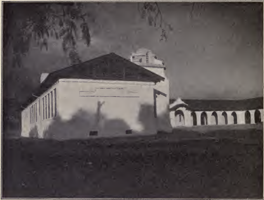
Santa Paula Grammar School. A practical adaptation of the old Spanish colonial architecture.
