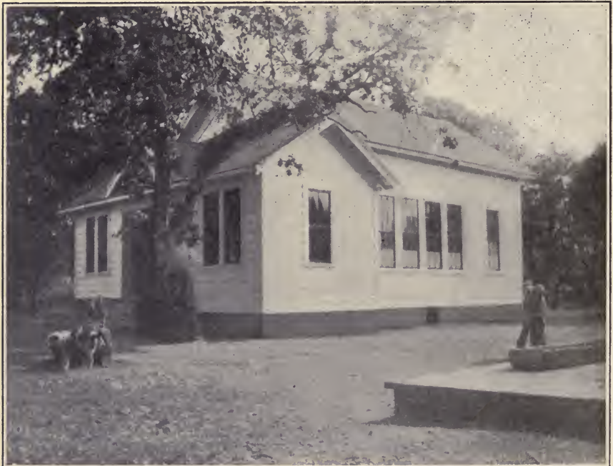
Remodeled Mill Creek School in Mendocino County, showing what can be done in many country districts.
