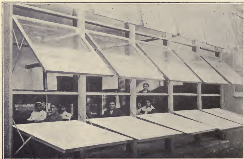
Interior of Hacienda School, showing open-air features.
