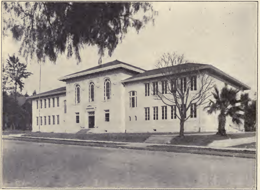
Wild Rose Grammar School at Monrovia. Good handling of a two-story building.
