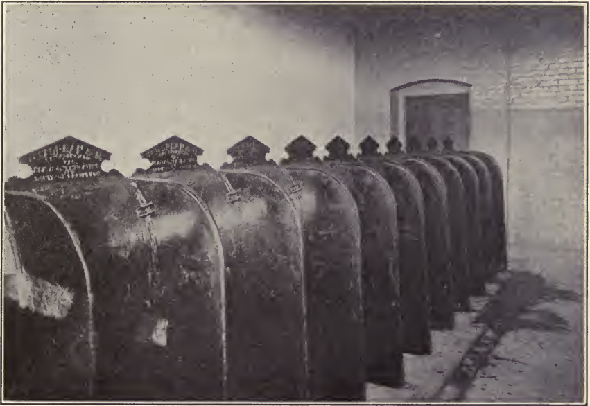
Objectionable latrine urinals with cast iron stalls. Out of date.
