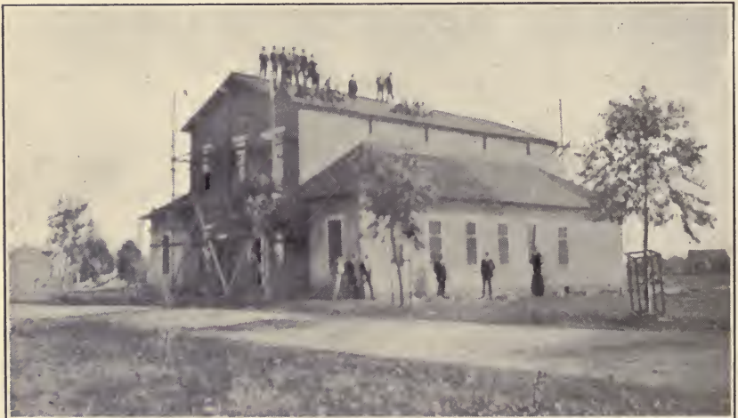
Red Bluff Manual Training Building in its final form, 52 by 60, cost $2,000. All work done by the boys.
