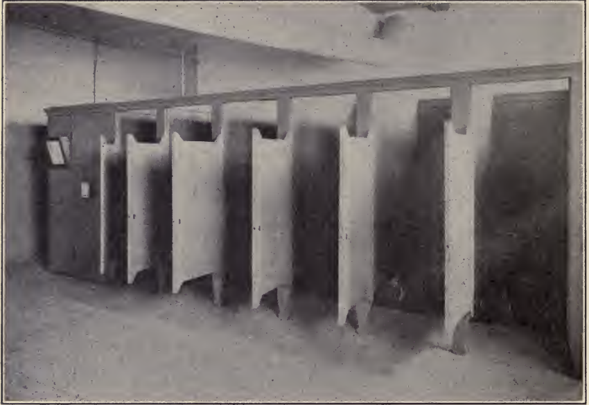
Objectionable and obsolete latrine toilet. Should be discarded.
