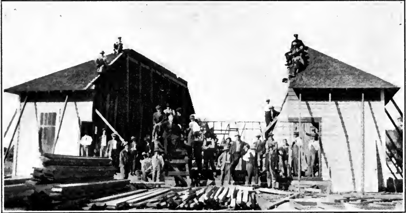
Red Bluff Manual Training Building. Splitting its shell for the third transformation. A genuine piece of work by the boys.
