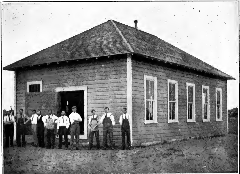
Red Bluff Manual Training Building, as originally built by the boys. Size 24 by 40, cost $600
