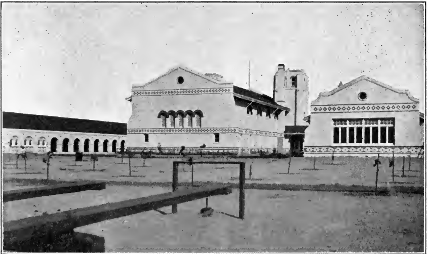
Rear view of the Lincoln Grammar School at Madera. Observe the fine effect of design in red bricks against a white background of cement bricks.
