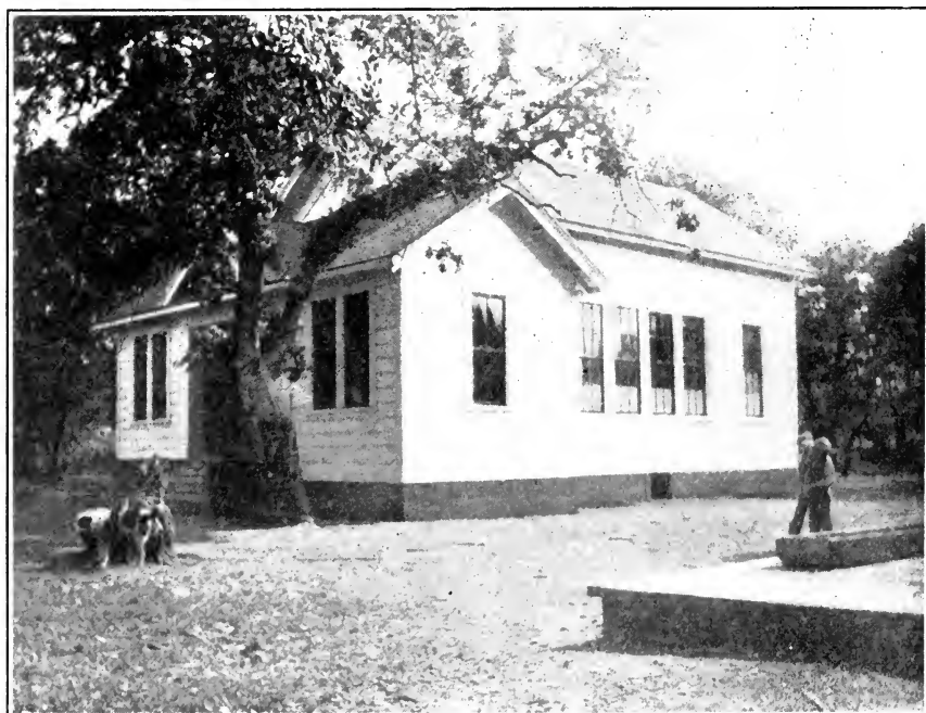
Remodeled Mill Creek School in Mendocino County, showing what can be done in many country districts.
