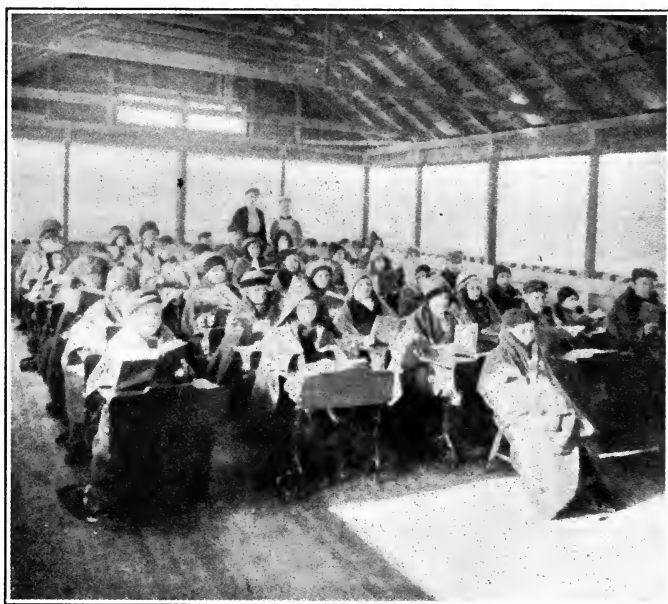
Open-air classroom in Massachusetts. Heat supplied by food and confined by hoods and blankets.
