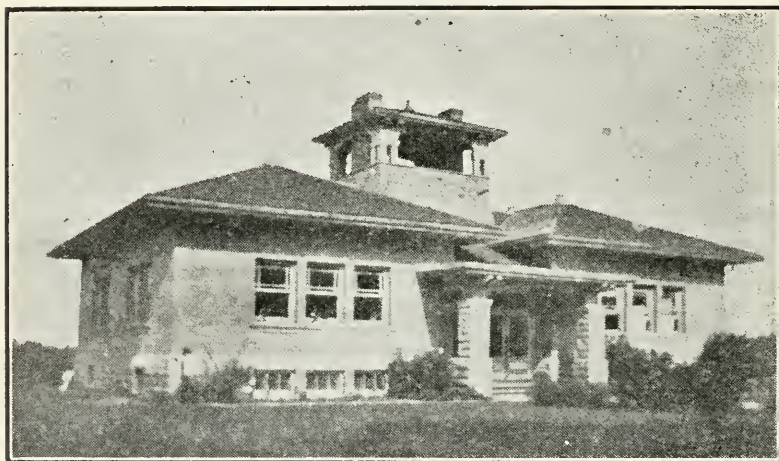
AN ONTARIO RURAL SCHOOL, KIRKFIELD, VICTORIA COUNTY There is a playground of three acres.
