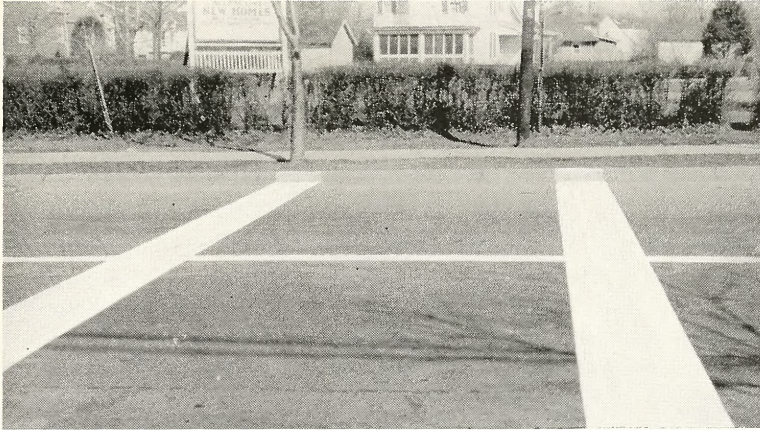
Fig. 12. At mid-block crossings, crosswalks should have lines at least two feet wide to be easily visible to motorists.
