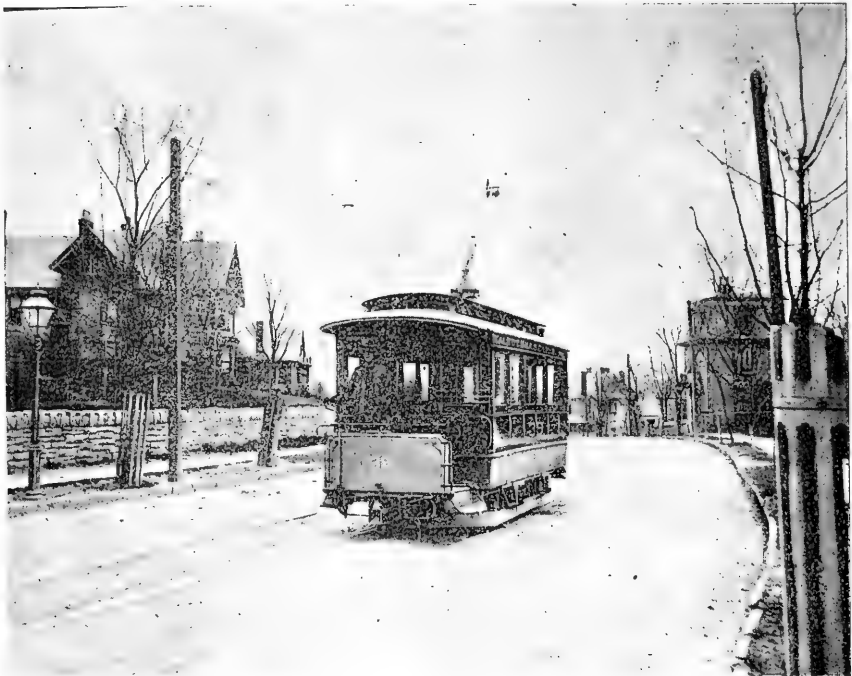
DAFT ELECTRIC ROAD, CINCINNATI, ROUNDING CURVES.
