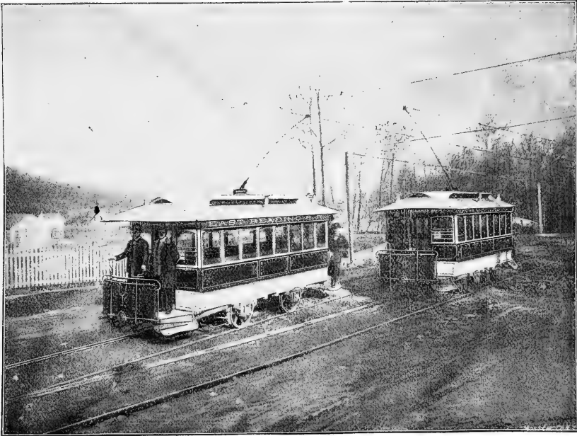
TURNOUT ON THE SPRAGUE ELECTRIC ROAD AT READING, PENN.
