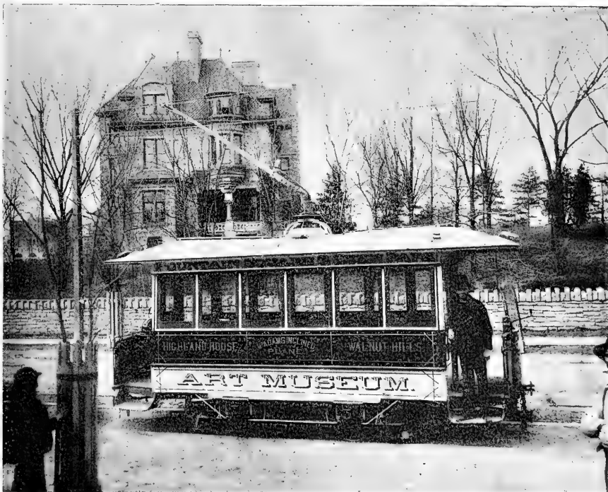
DAFT ELECTRIC ROAD, WALNUT HILLS, CINCINNATI.
