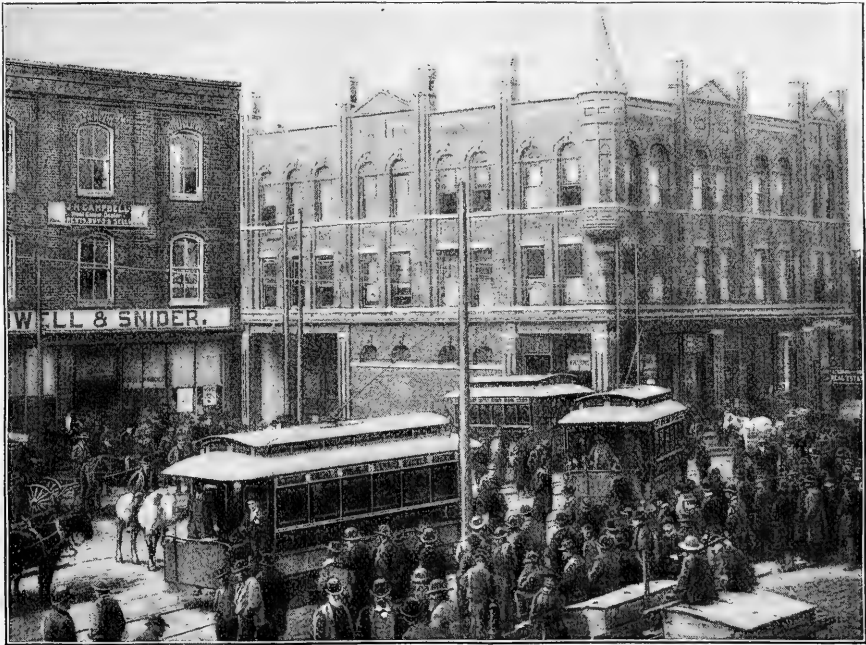
VIEW OF ELECTRIC ROAD AT ASHEVILLE, N.C.
