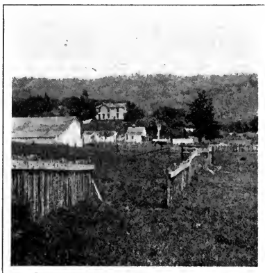
FENCE BROKEN BY SLIPPING OF THE EARTH ALONG A FAULT LINE.
