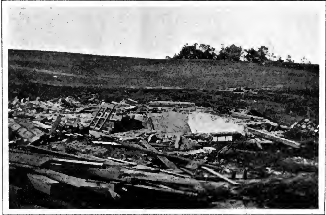
REMAINS OF FARM BUILDINGS DESTROYED BY A TORNADO.
