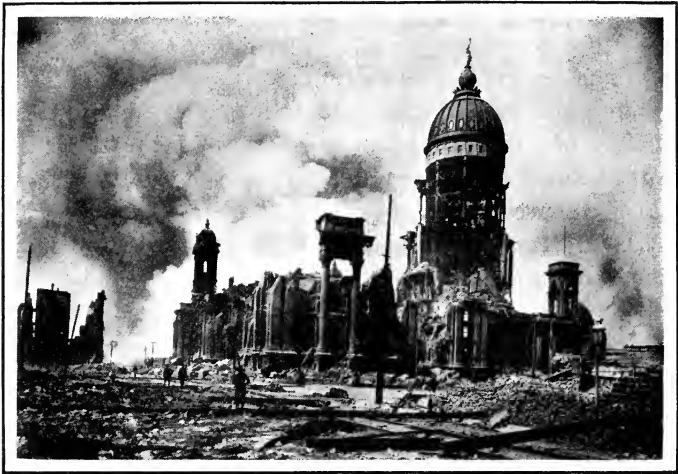
THE RESULT OF AN EARTHQUAKE.
