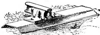
Metal Track, London and Northwestern Railway of England, A. D. 1889.
